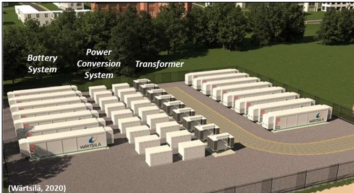
Figure 8: Pivot Power's proposed 50MW lithium-ion battery in Kemsley, Kent.
