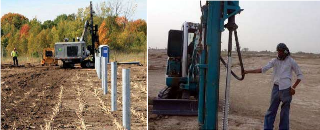
Figure 7: Driven/ Rammed Steel Pile (left) and Ground Screw (right) are the preferred mounting technology.
