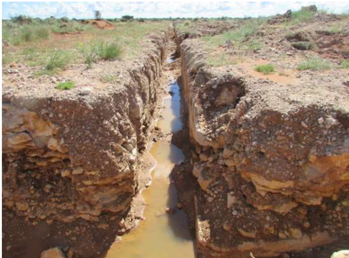
Figure 9: One of the old trenches filled with water from recent rains.
