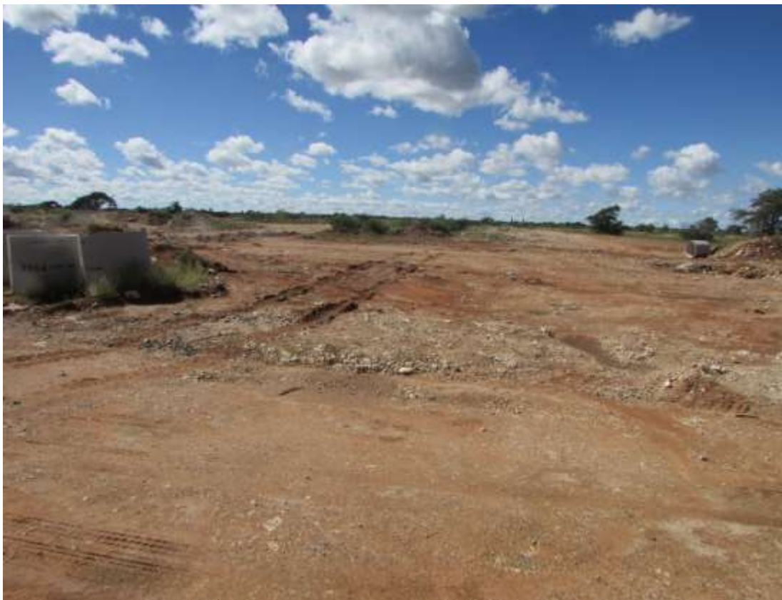
Figure 5: Another part of the area where work is ongoing.
