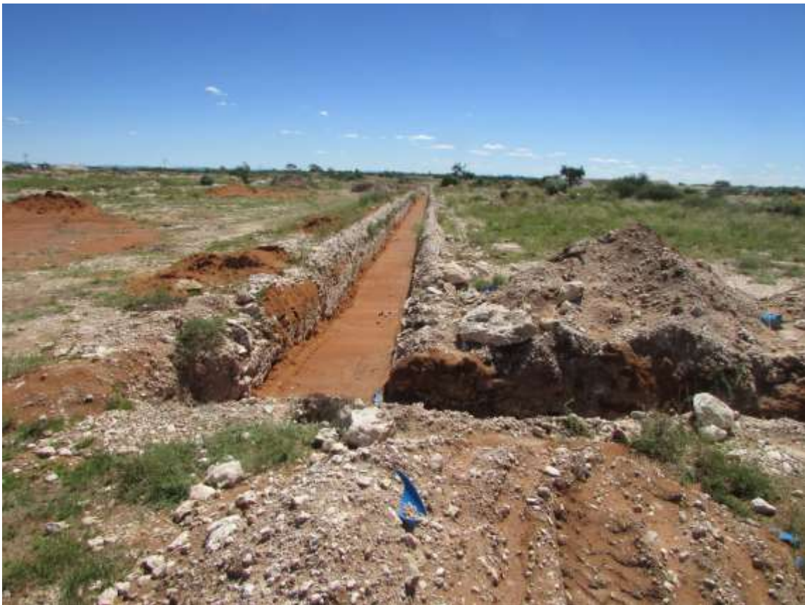
Figure 15: Area where trenches have been partially back-filled and compacted.
