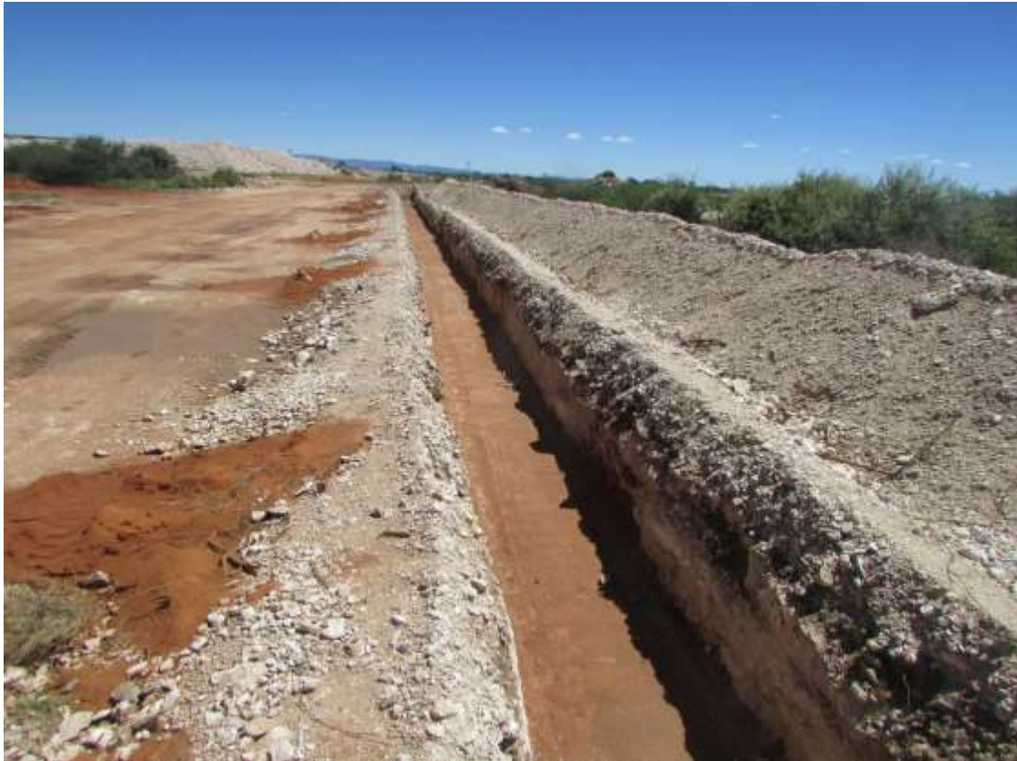
Figure 14: Recently excavated trenches.
