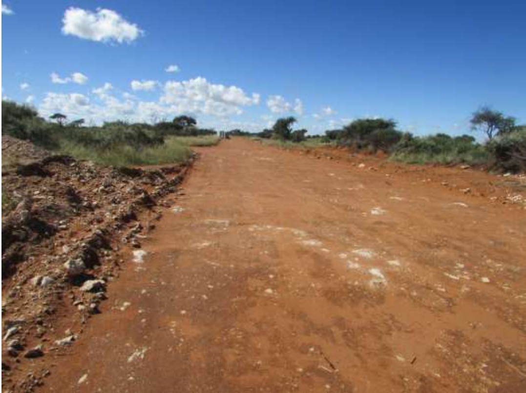
Figure 6: One of the internal roads that have been scraped & compacted.
