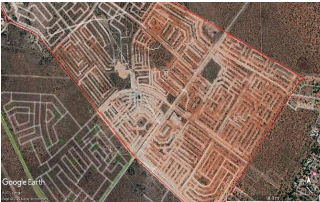
Figure 3: A closer view of the study & development area in March 2022 showing the extent of the earthworks related to the installation of services (sewerage, water pipelines & internal road networks) (Google Earth 2022).
