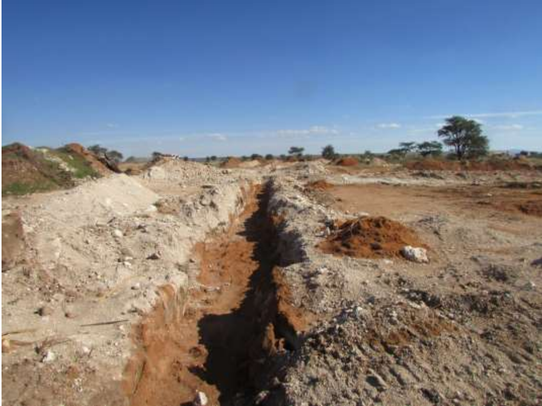
Figure 7: The trenches and soil/waste rock dumps around the Locality 1.
