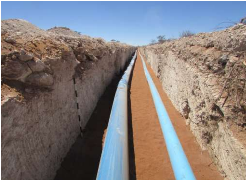
Figure 65: Another view of Trench 3.
