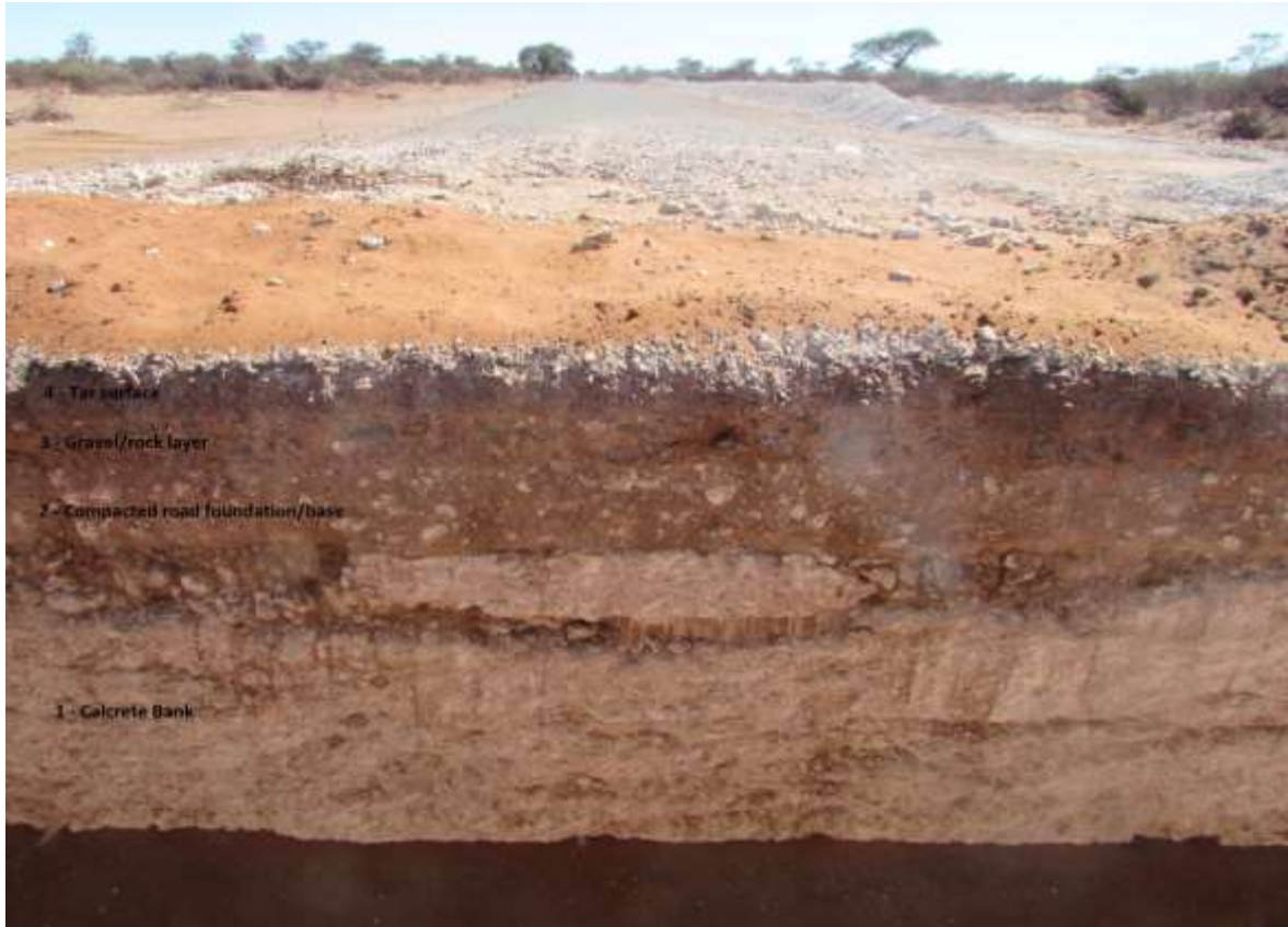
Figure 25: Trench through northern section of tar road.
