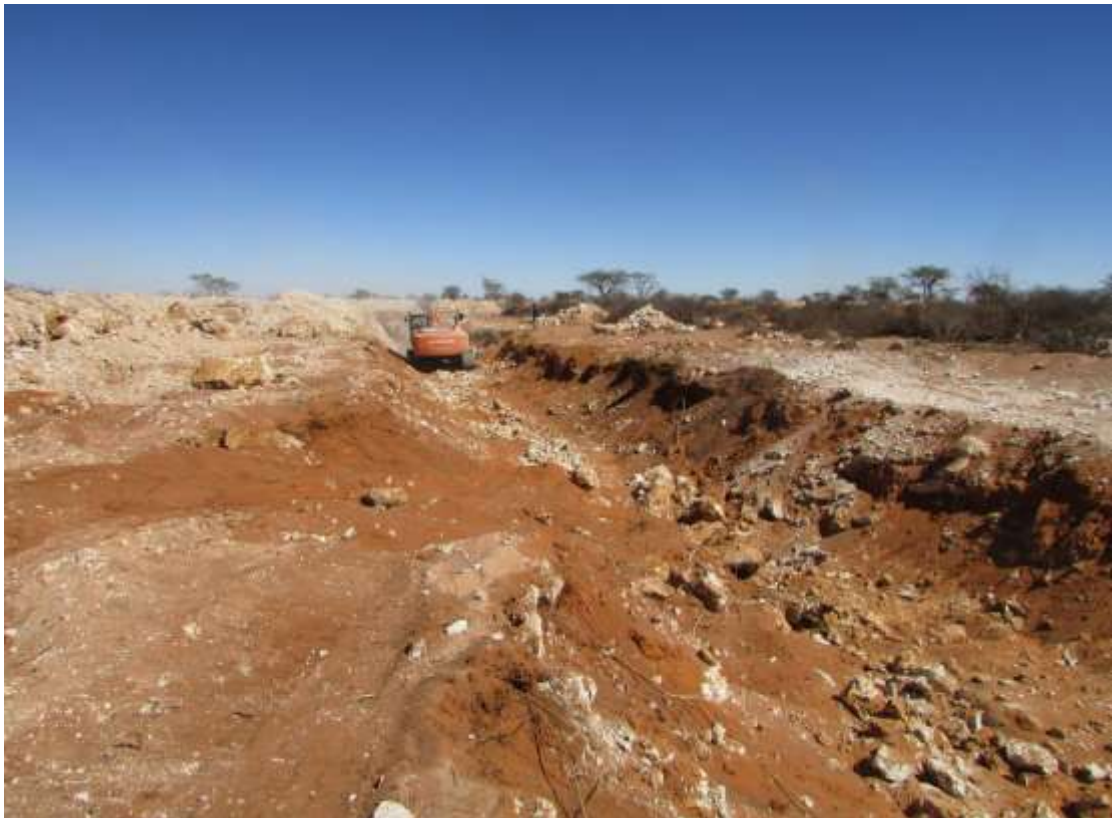
Figure 61: Another section of the trench with ongoing work visible.
