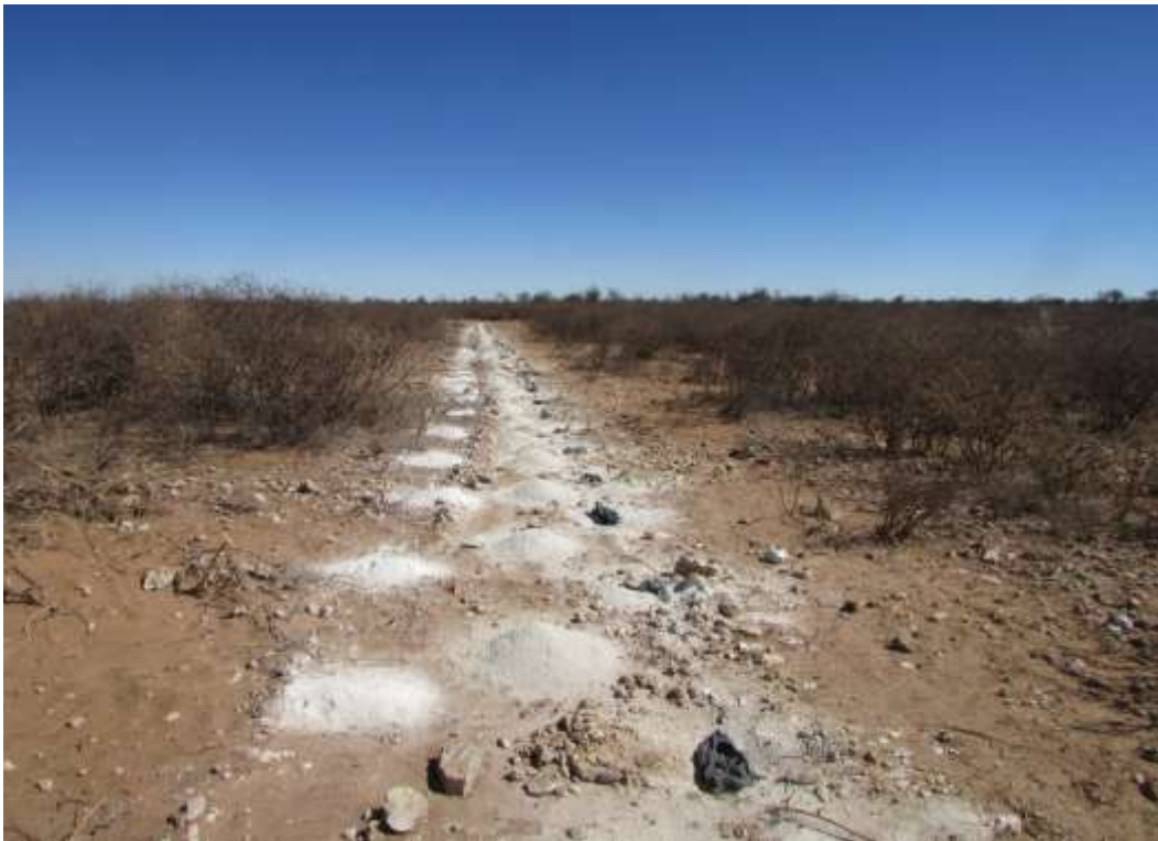
Figure 37: An area prepared for blasting.
