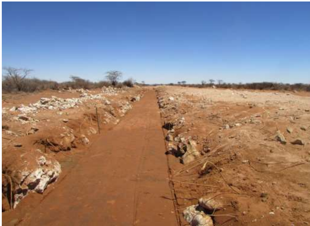
Figure 67: Another section of Trench 4.
