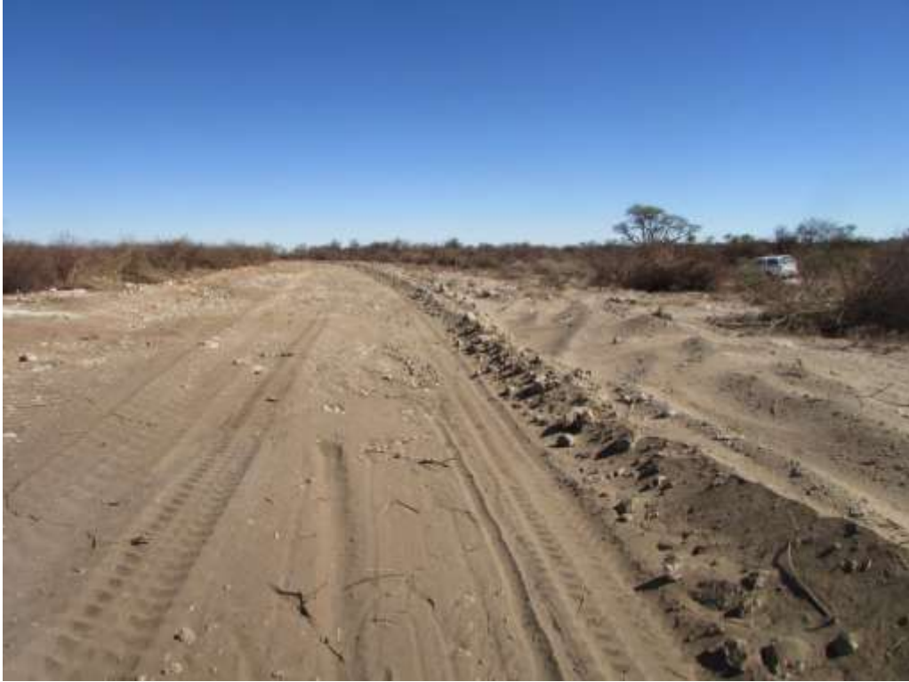
Figure 36: One of the new roads in the area.
