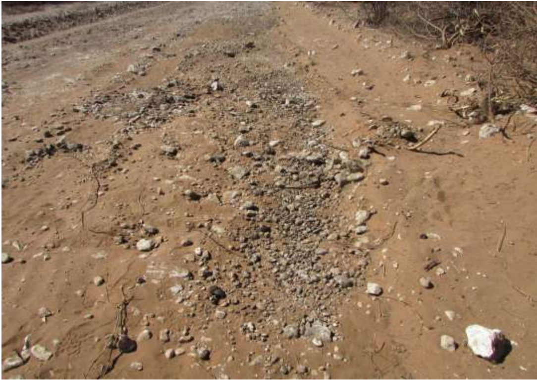
Figure 38: Close-up of new road surface after grading.
