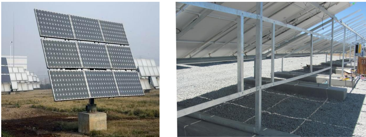
Figure 8 & 9: Examples single axis & fixed solar cast foundations.
