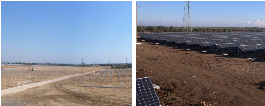
Figures 20 & 21: Typical internal road and track examples (Source: Solek Engineering Report, 2012).
