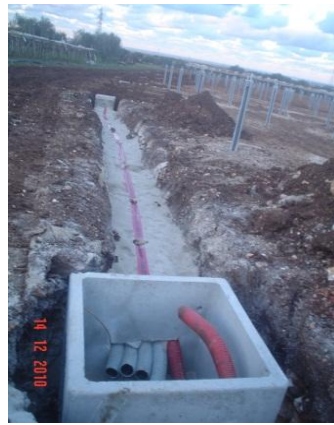
Figures 16, 17 & 18: Photos of typical underground cable trenches (Source: Solek Engineering Report, 2012).
