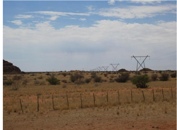
Figure 23: Existing 132kV power line, north of solar site.
