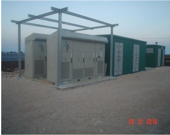
Figures 14 & 15: Typical examples of on-site step-up substations (Source: Solek Engineering Report, 2012)
