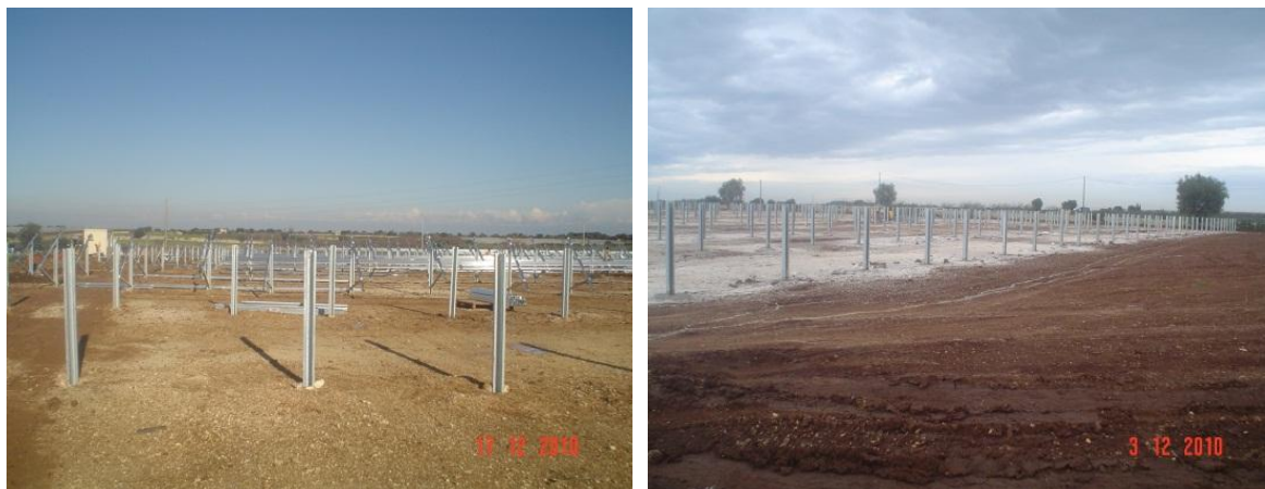
Figure 19: Example of foundation structures – rammed piers/poles.
