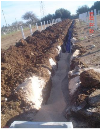
Figures 16, 17 & 18: Photos of typical underground cable trenches (Source: Solek Engineering Report, 2012).
