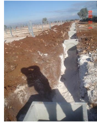
Figures 16, 17 & 18: Photos of typical underground cable trenches (Source: Solek Engineering Report, 2012).
