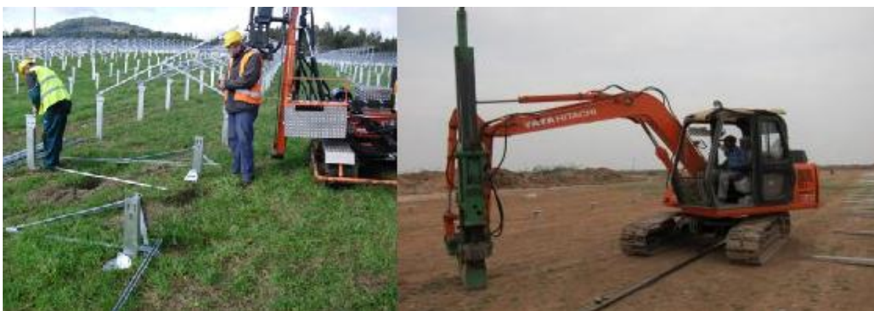
Figures 10 & 11: Ramming equipment for solar mounting structures (Source: Solek Layout Report, 2012).
