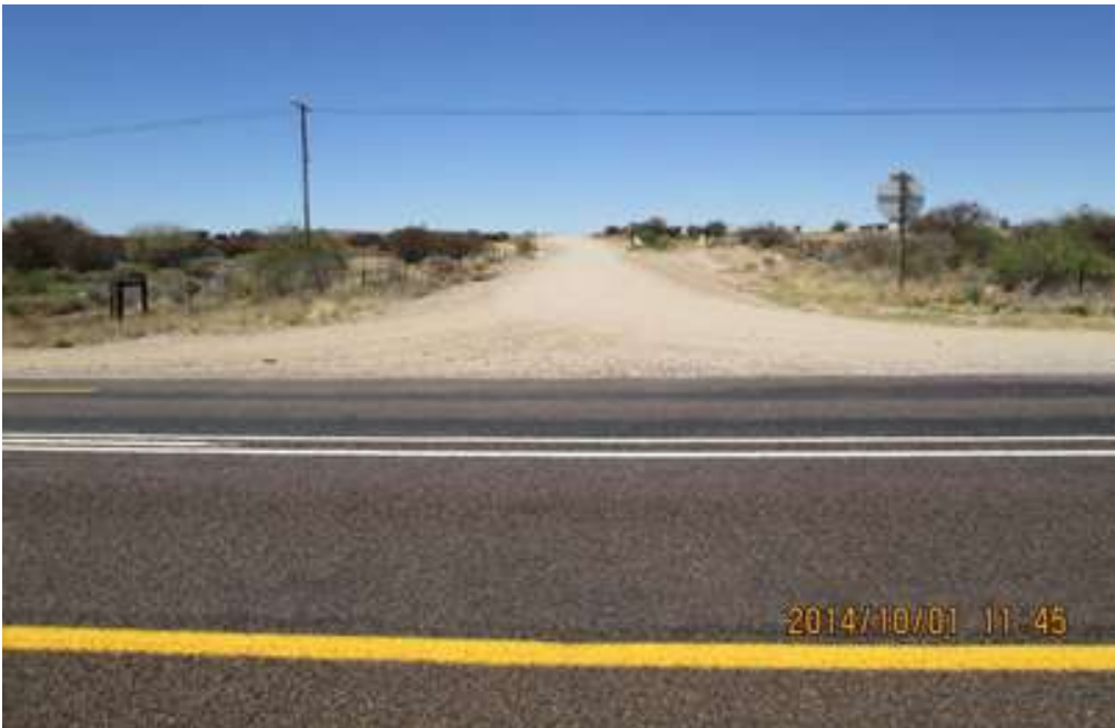
Figure 32: N10 / Kleinbegin intersection
