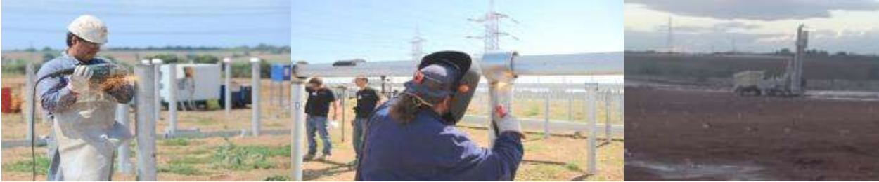
Plate 9: Showing typical erection of Solar PV modules
