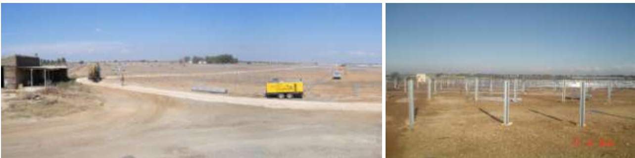
Plate 8: Typical example of site preparation activities (Solek, 2014)
