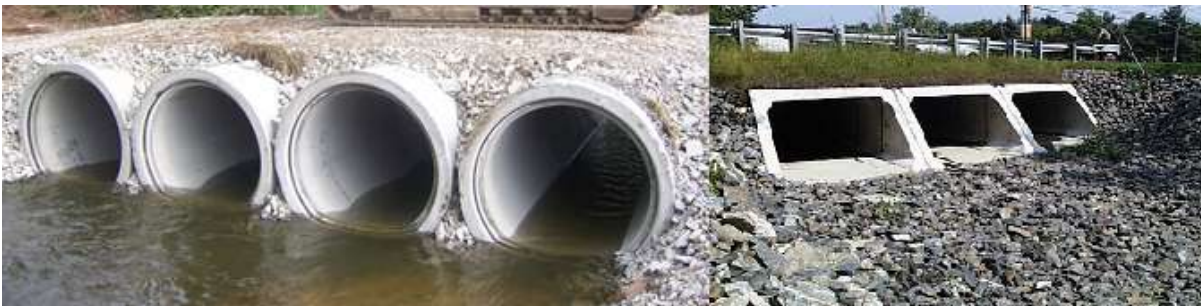
Figure 22: Installed concrete pipes and culverts
