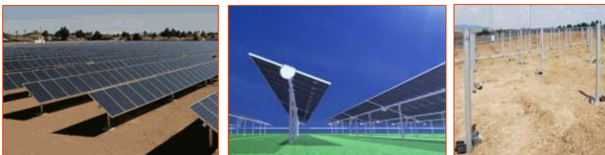
Plate 1: Examples of various mounting alternatives (Solek, 2014)
