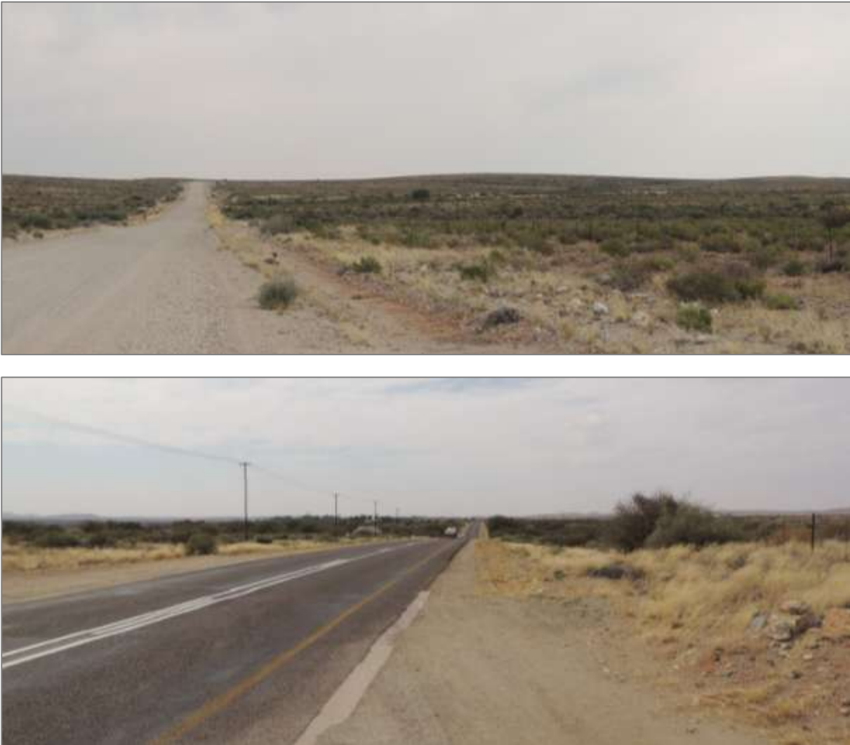
Figure 51: Photograph taken of the N10 (bottom) and Klienbegin (top) roads
