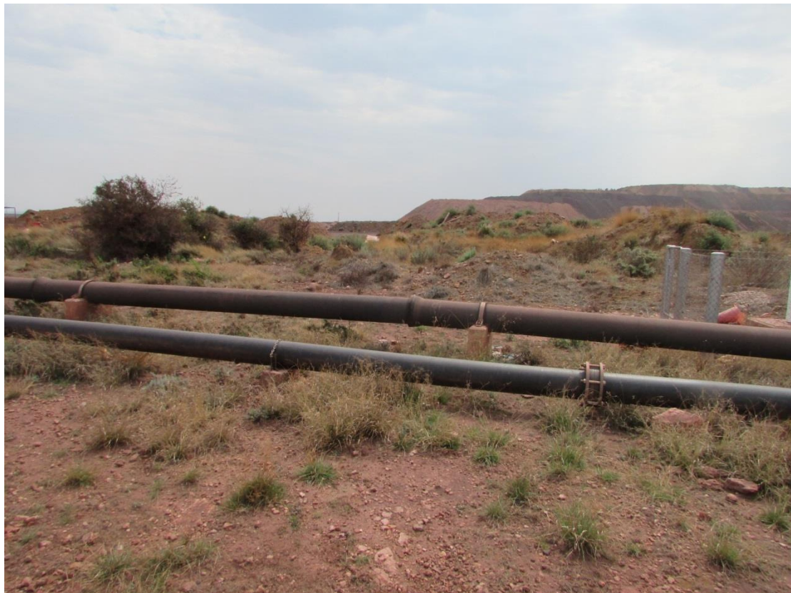
Figure 10: A view of the general area close to the original KOL 6 pan site.
