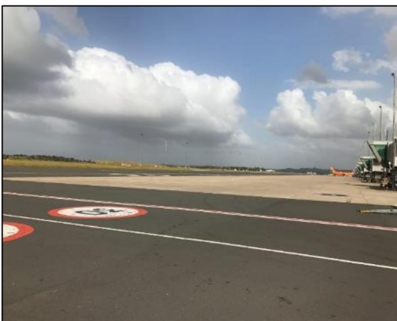
Photo 11: Facing SW from GSE parking, showing existing alpha apron
