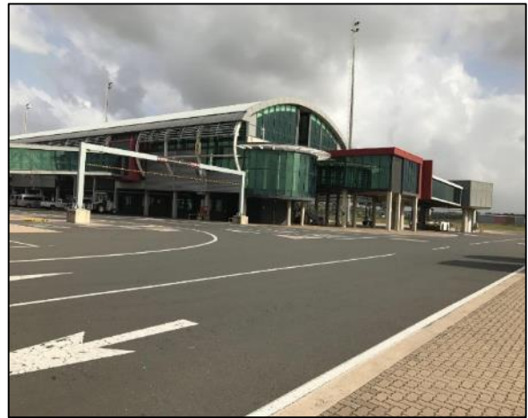
Photo 10: Facing W from GSE parking, showing existing terminal
