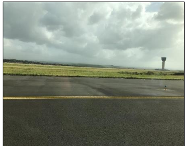
Photo 6: Facing North (N) from existing Taxiway Bravo showing control tower in background
