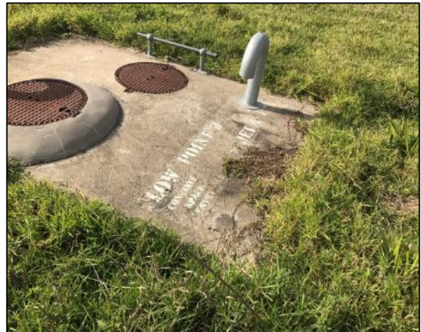
Photo 26: Stormwater infrastructure on the proposed site of remote apron stands
