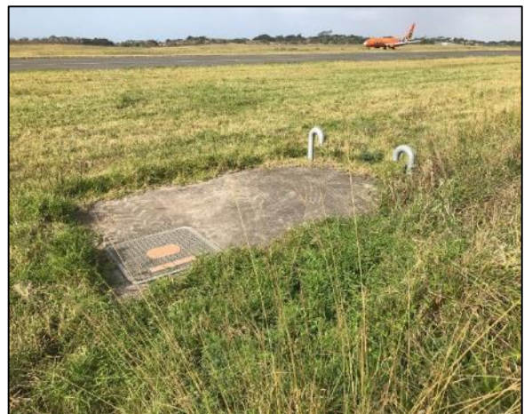
Photo 28: Facing SE from the proposed site of remote apron stands (between new Taxiways Foxtrot and India), stormwater infrastructure visible, existing taxiway bravo in background
