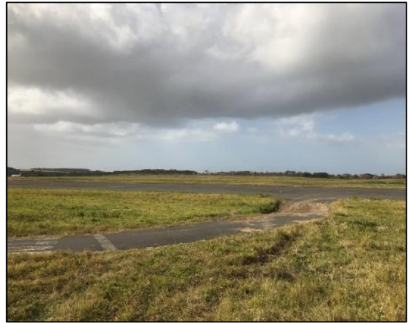
Photo 4: Facing East (E) from link road off existing taxiway bravo, showing existing taxiway bravo (site of proposed remote concrete apron stand)
