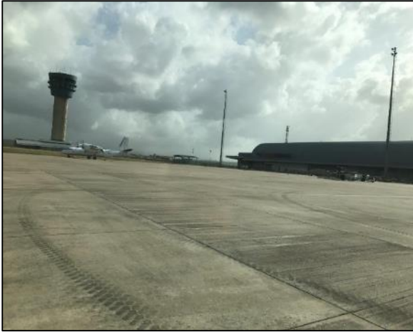
Photo 1: Facing North (N) from Delta Apron, with control tower in view
