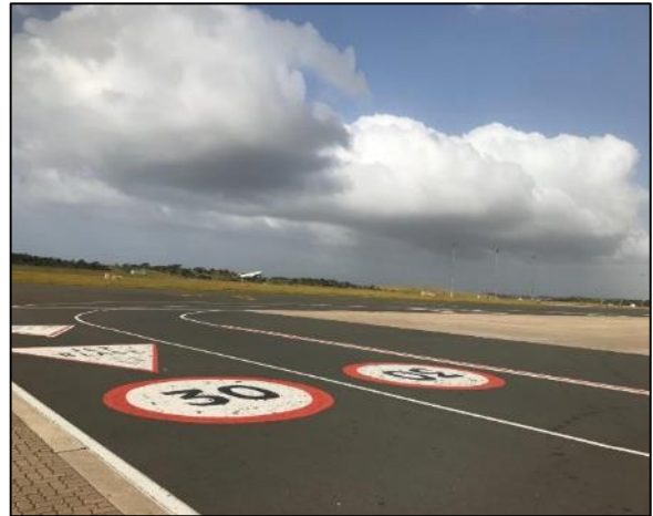
Photo 8: Facing South (S) from GSE parking, adjacent to existing taxiway F and showing apron stands
