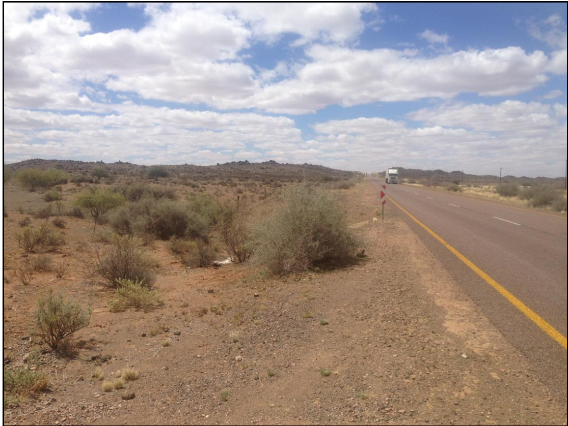
Figure 6: The R27 arterial road.
