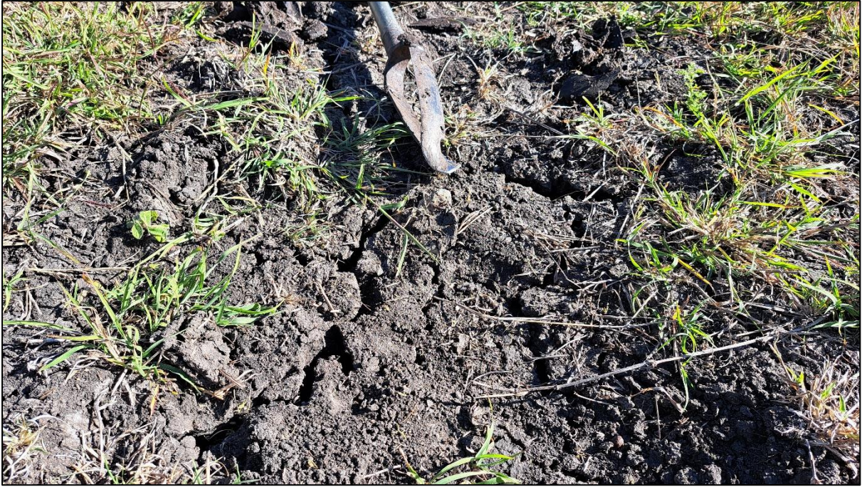
Figure 8: Vertic topsoil swelling and shrinking which causes self-plough or cracking (TBC1, 2023)
