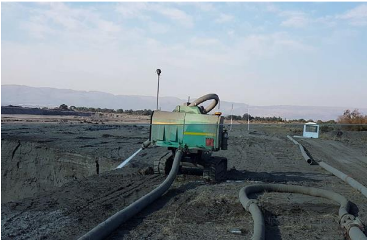
Figure 4: Example of hydraulic re-mining of a tailings dam facility
