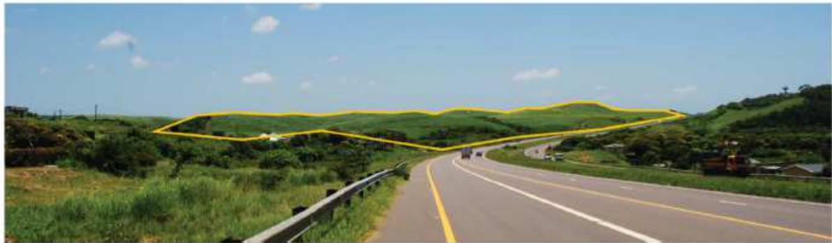
Figure 3-72: View Point 8 - View from the N2, looking north. The site is highly visible from this point.
