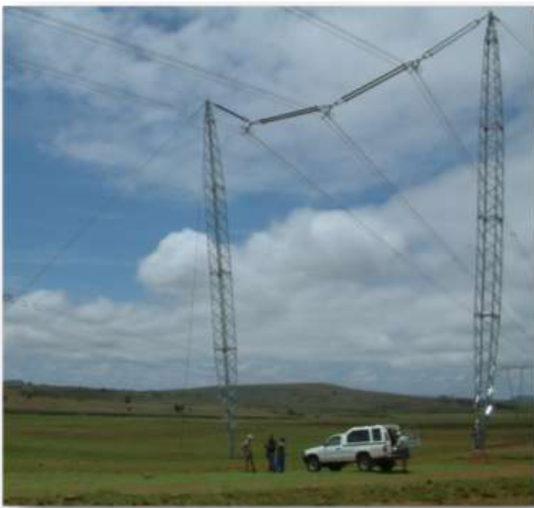
Plate 2: Cross Rope Tower
