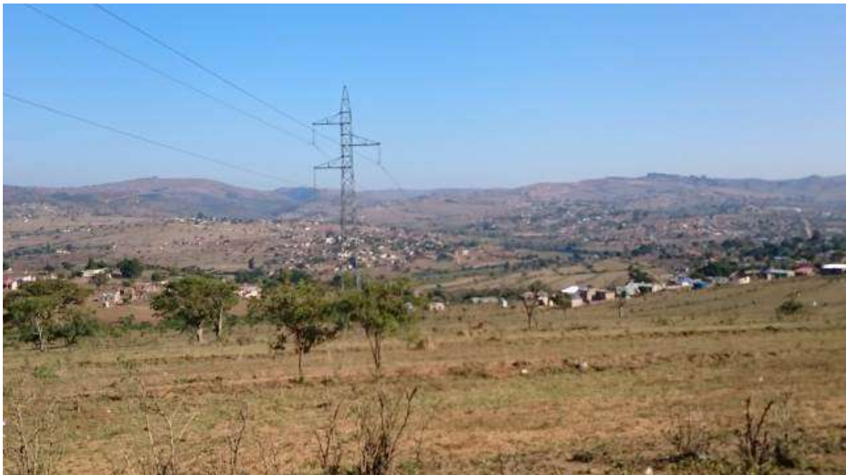
Plate 6: Corridors in Section A-B adjacent to the N2
