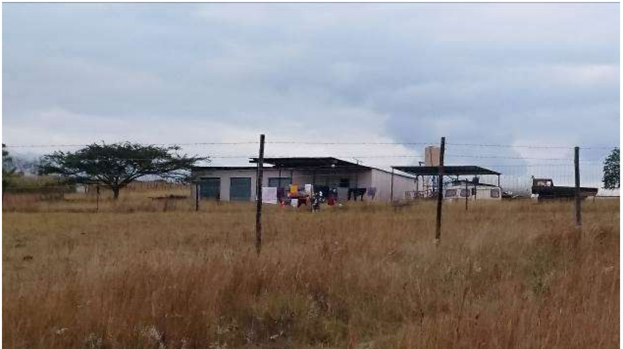
Plate 10: Dwelling in corridor AE
