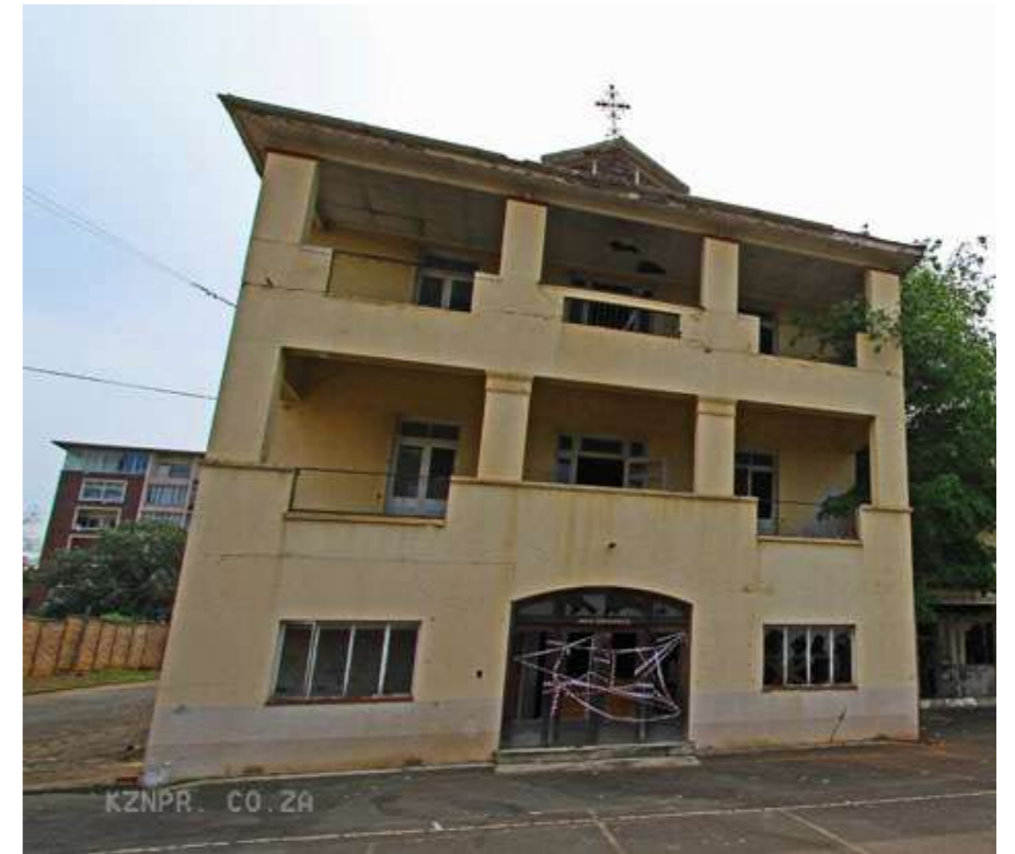
BLOCK A / EXTERIOR
