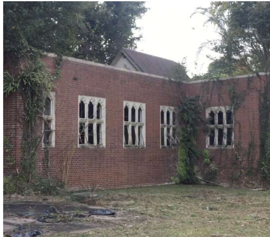
BLOCK E / CHAPEL / EXTERIOR
