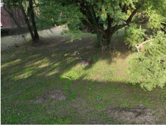
Photo 9 : Showing overflow of sewer discharge at sewer manhole located at the bottom of earth bank.
