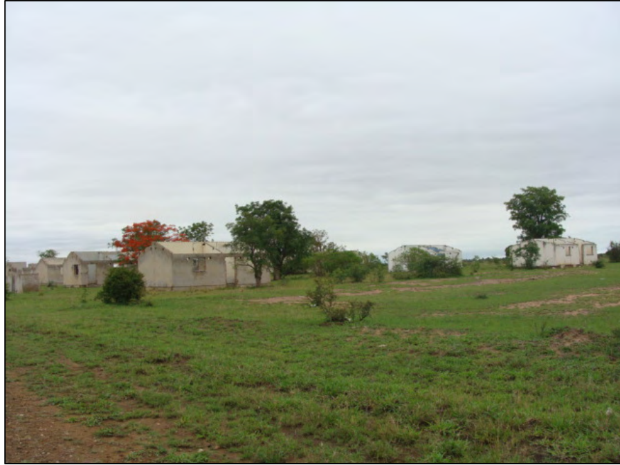
Figure 27: Derelict buildings at Site 1.
