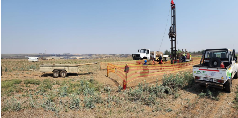
Figure 6: Barricaded site (Yellow & red safety net).
