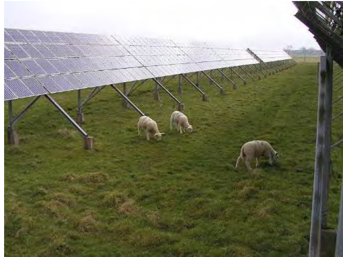
Figure 3.10: PV ground mounted system 20
