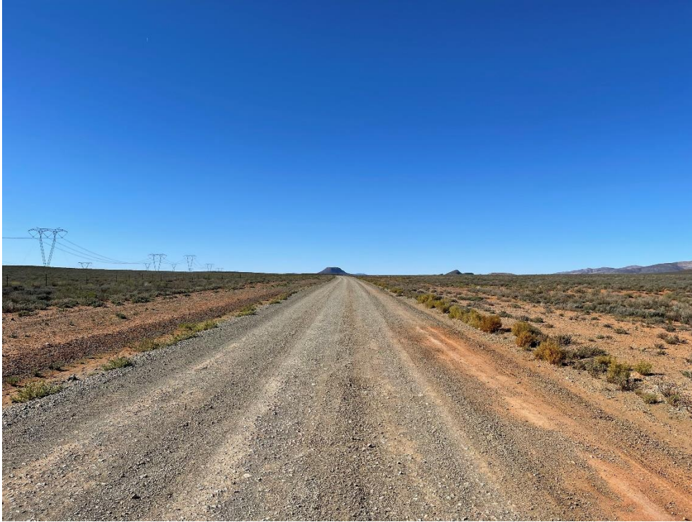
Figure 7.6 Existing Road OP06121 –East Approaching
