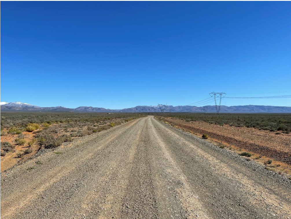
Figure 7.5 Existing Road OP06121 – West Approaching
