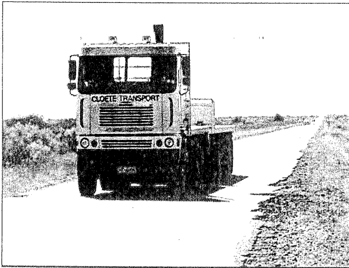
Figure 3-32: Vehicle shying away from edge break
