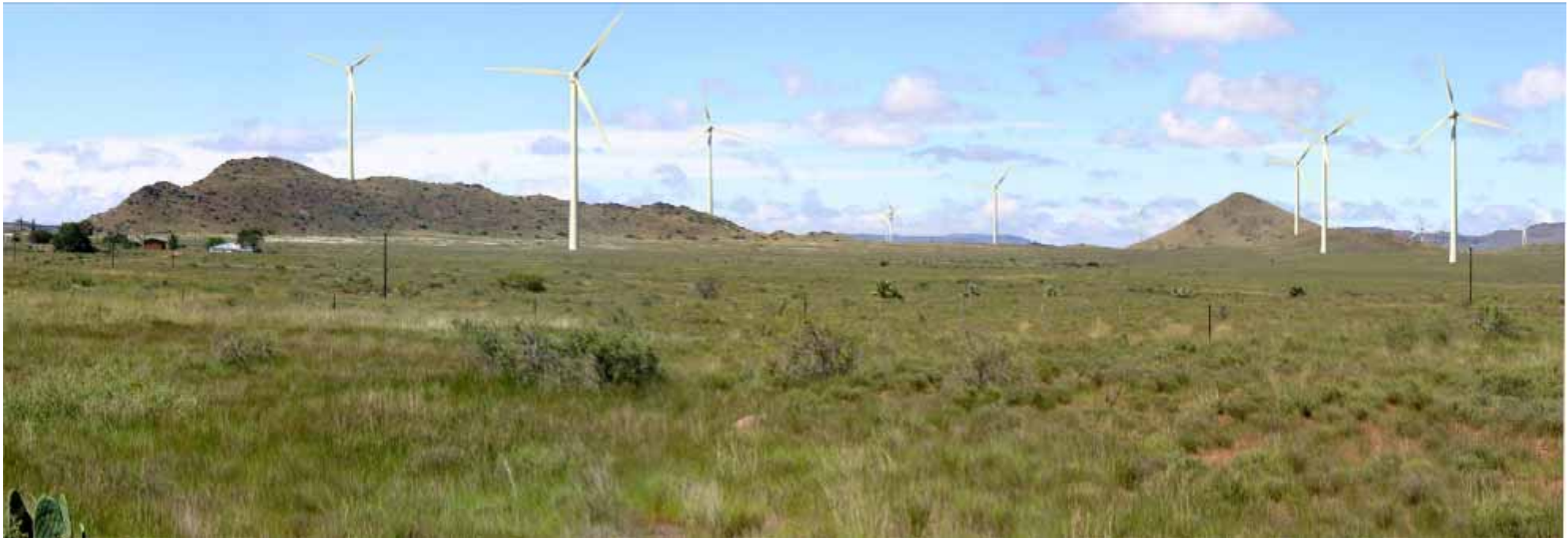
Figure 6.10: Post construction panoramic overview from representative of a short distance visual experience that travellers, residents, farmers, commuters (using the train) and potential tourists utilising the area around the Biesiespoort Substation will have of the facility.
