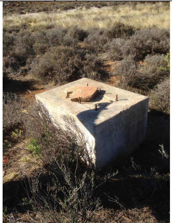
Photo 38. Existing municipal borehole VBH06.
