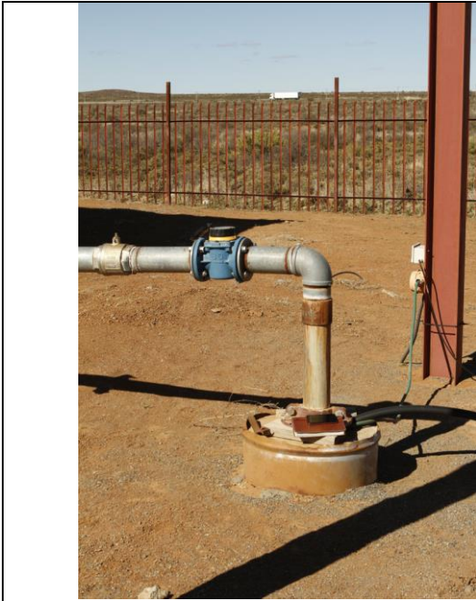
Photo 39. Existing municipal borehole VBH07.
