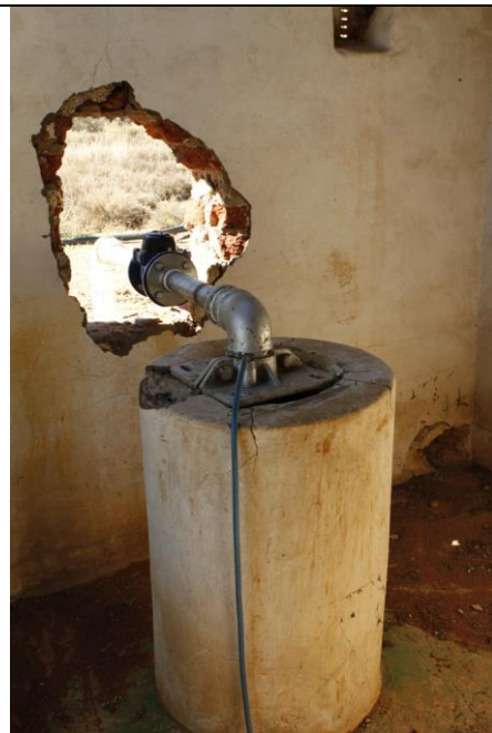
Photo 34. Existing municipal borehole VBH02.
