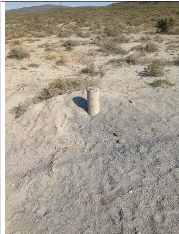
Photo 23. Newly drilled borehole HBH08 (HP01).
