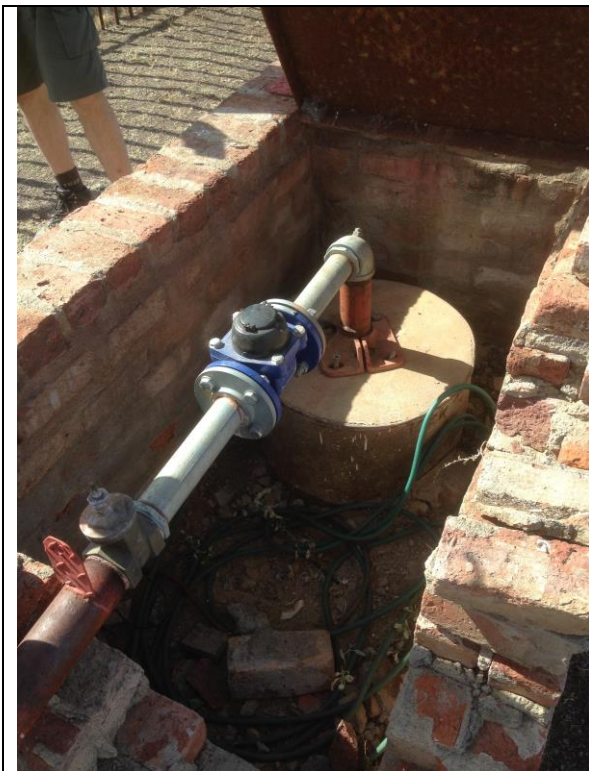
Photo 52. Existing municipal borehole RBH01.
