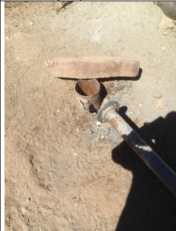
Photo 44. Existing municipal borehole BH-BK04.
