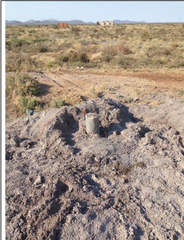
Photo 25. Newly drilled borehole HBH09 (HP03).
