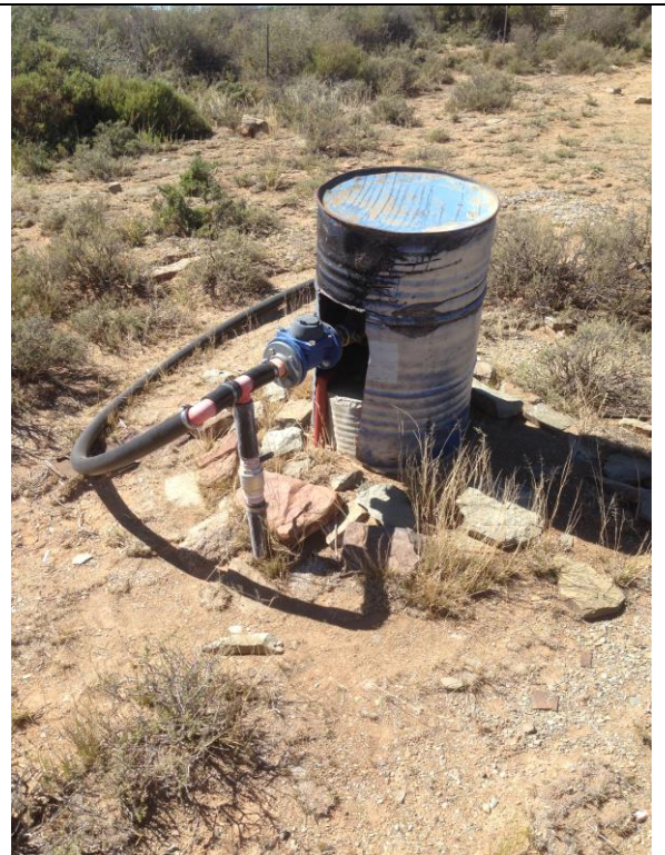
Photo 41. Existing Municipal Borehole BH-BK01.
