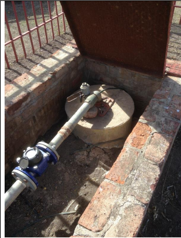
Photo 54. Existing municipal borehole RBH03.
