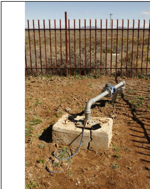
Photo 33. Existing municipal borehole VBH01.
