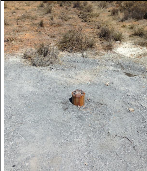
Photo 29. Newly drilled borehole MBH02 (MP01).
