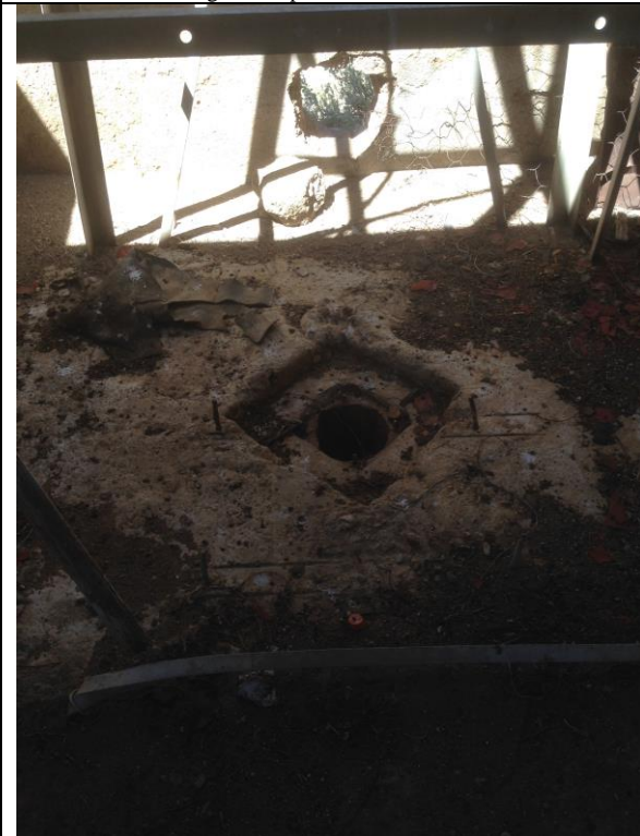
Photo 48. Existing municipal borehole BH-WP01.
