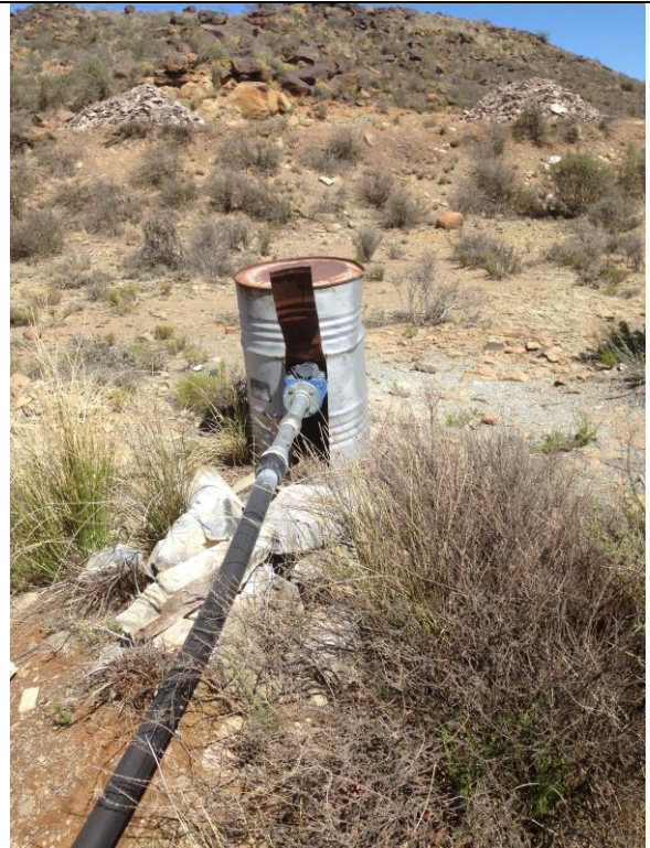
Photo 43. Existing municipal borehole BH-BK03.
