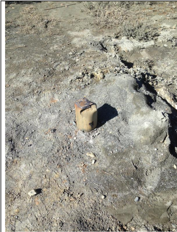
Photo 1. Newly drilled borehole VBH08 (VWP01).
