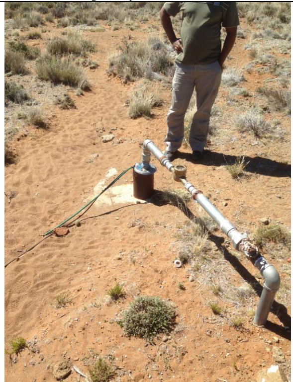
Photo 45. Existing municipal borehole BH-BK05
