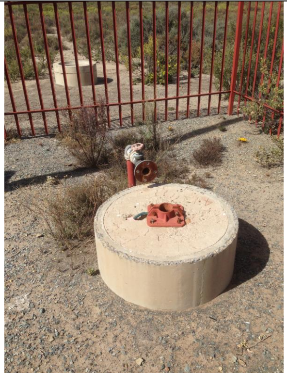
Photo 55. Existing municipal borehole RBH04.
