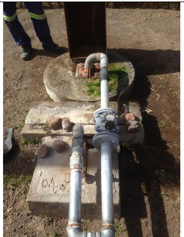
Photo 53. Existing municipal borehole RBH02.
