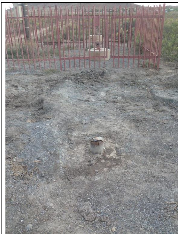
Photo 21. Re-drilled municipal production borehole RBH04.
