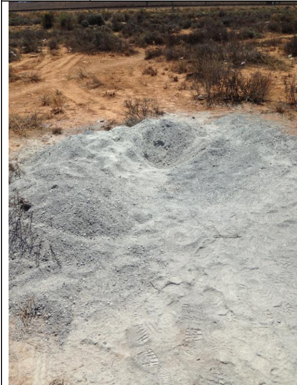
Photo 31. Newly drilled borehole MP02.
