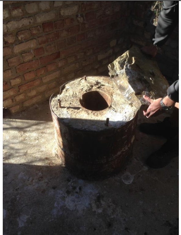
Photo 36. Existing municipal borehole VBH04.
