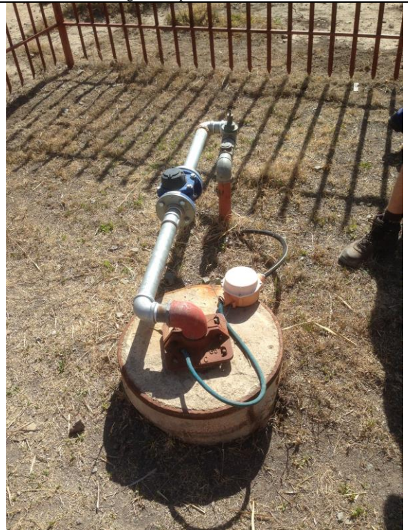
Photo 57. Existing municipal borehole RBH06.
