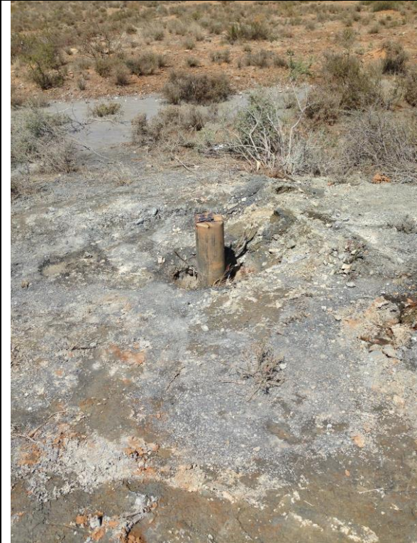
Photo 7. Newly drilled borehole VBH11 (VWP05).
