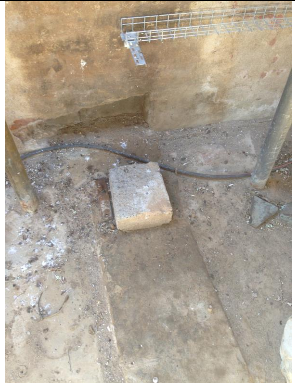
Photo 47. Existing municipal borehole BH-KG.
