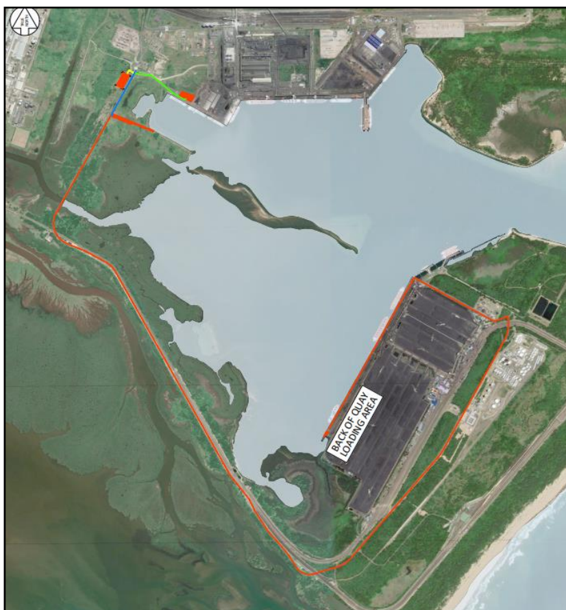
Figure 3-10: Existing access road to the proposed load-out berth
