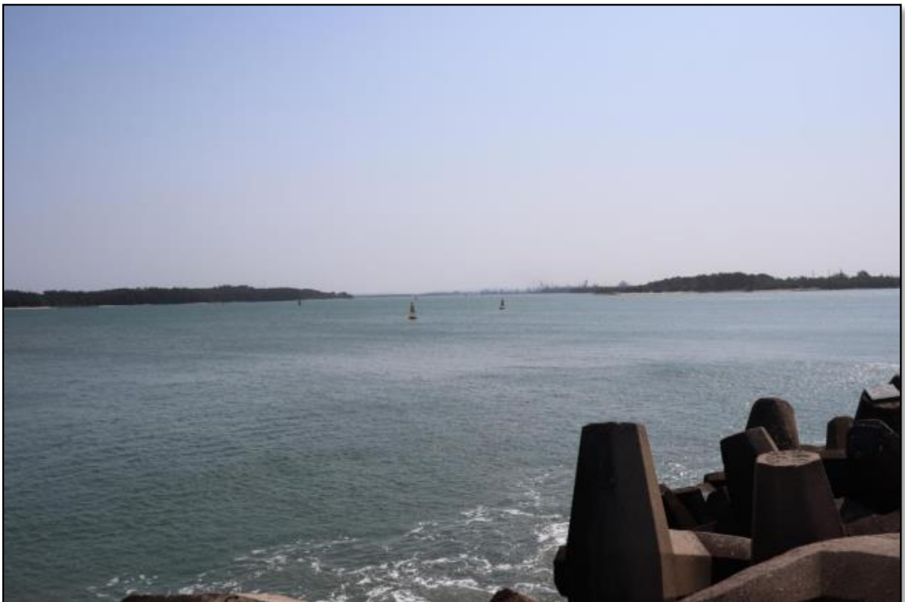
Figure 7-12: View from the Inner Northern Breakwater looking down the length of the Port.
