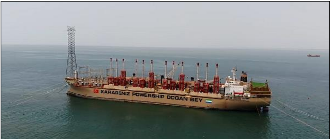
Figure 3-2: Powership mooring system.
