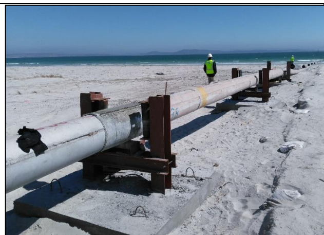
Figure 2-8 Typical Launchway across beach
