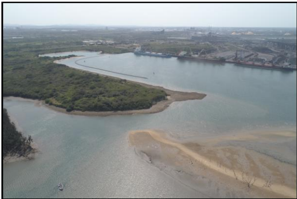
Figure 0-3: Overview of Port Site
