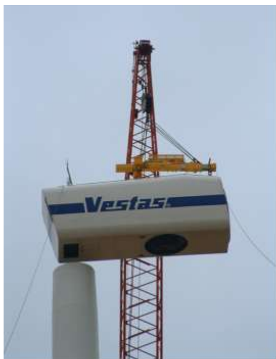
Figure 4.8: Photograph illustrating the assembly of a turbine (nacelle and blades) utilising a large lifting crane (photographs courtesy of Eskom from construction at the Klipheuwel demonstration facility)
