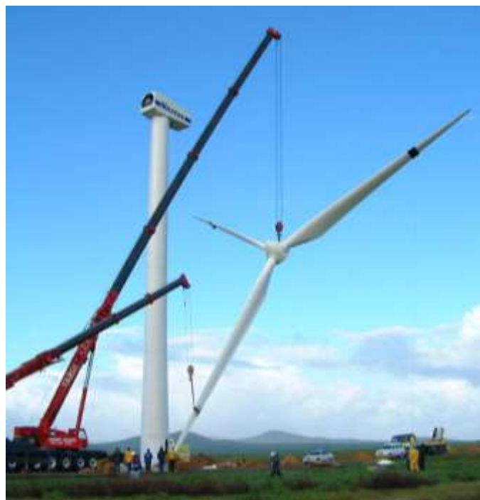
Figure 4.8: Photograph illustrating the assembly of a turbine (nacelle and blades) utilising a large lifting crane (photographs courtesy of Eskom from construction at the Klipheuwel demonstration facility)
