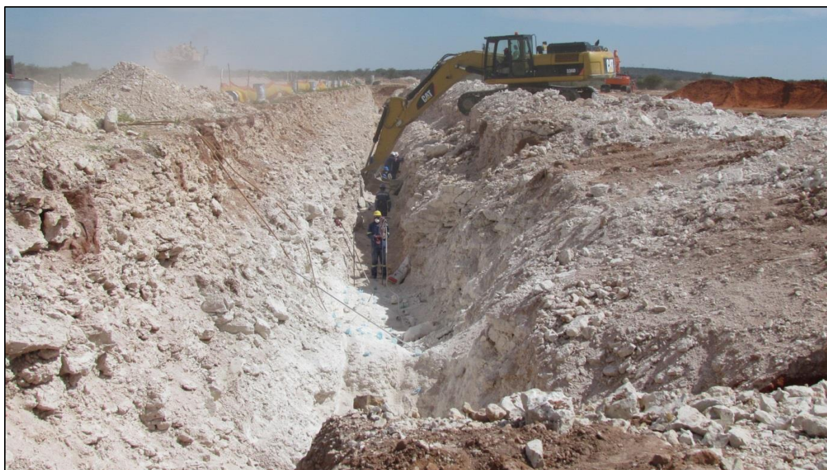
Fig. 4. Recent deep trenching within the Bestwood development area showing the thick development of calcrete hardpan in the subsurface (Image kindly provided by Dr D. Morris, McGregor Museum, Kimberley. January 2014).
