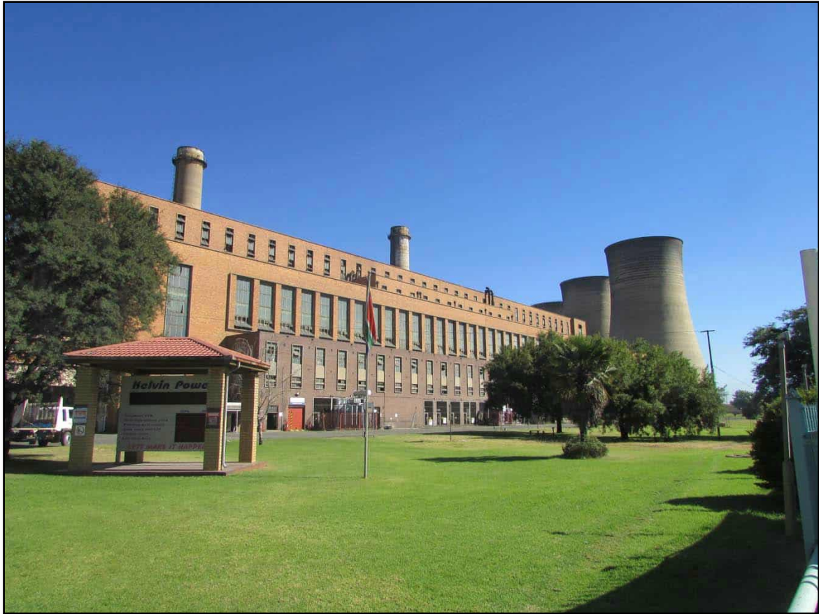
Figure 3: A view of A-Station and its Cooling Towers.
