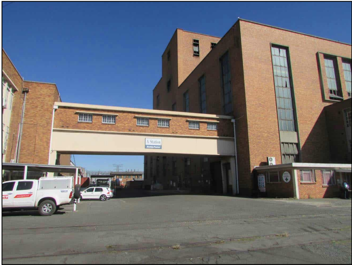
Figure 4: Closer view of A-Station and the “bridge” connecting it with Main Office Block & B Station.
