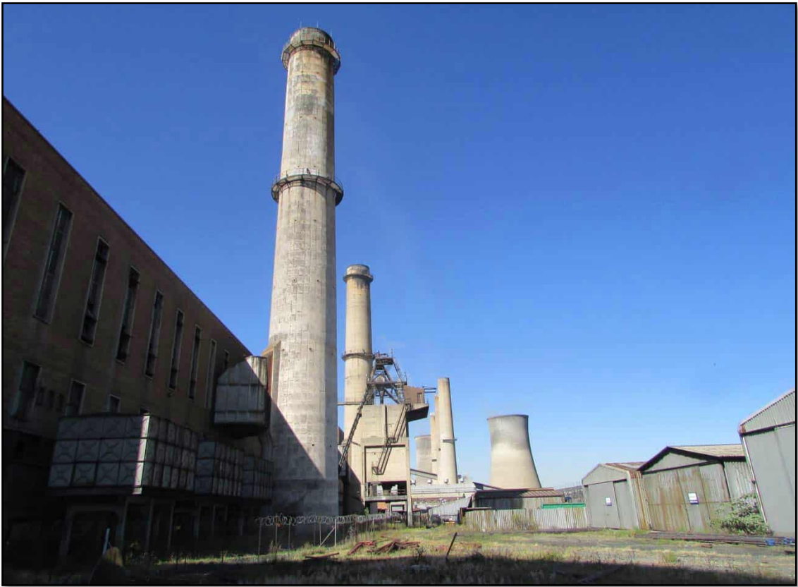
Figure 15: A view of the A-Station smoking stacks/towers looking towards B Station.
