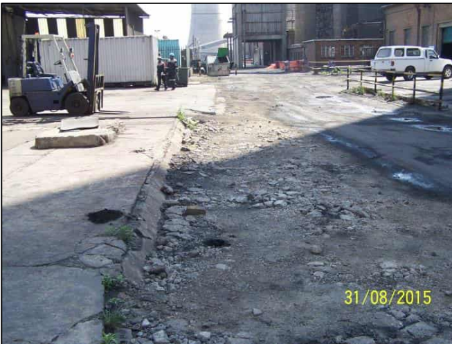
Figure 15: Surface of road along workshop area
