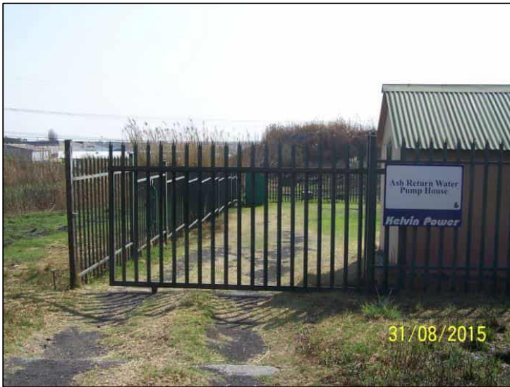
Figure 33: Pumphouse - Sample along southern fence
