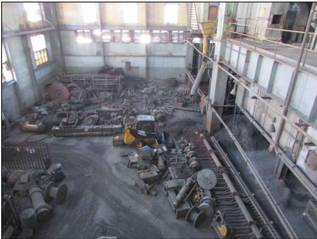
Figure 12: A view of some of the equipment and material in A-Station.
