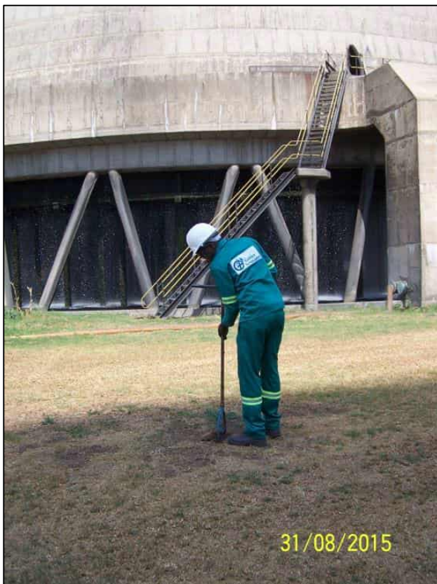
Figure 11: Position of Station B Cooling Towers auger sample
