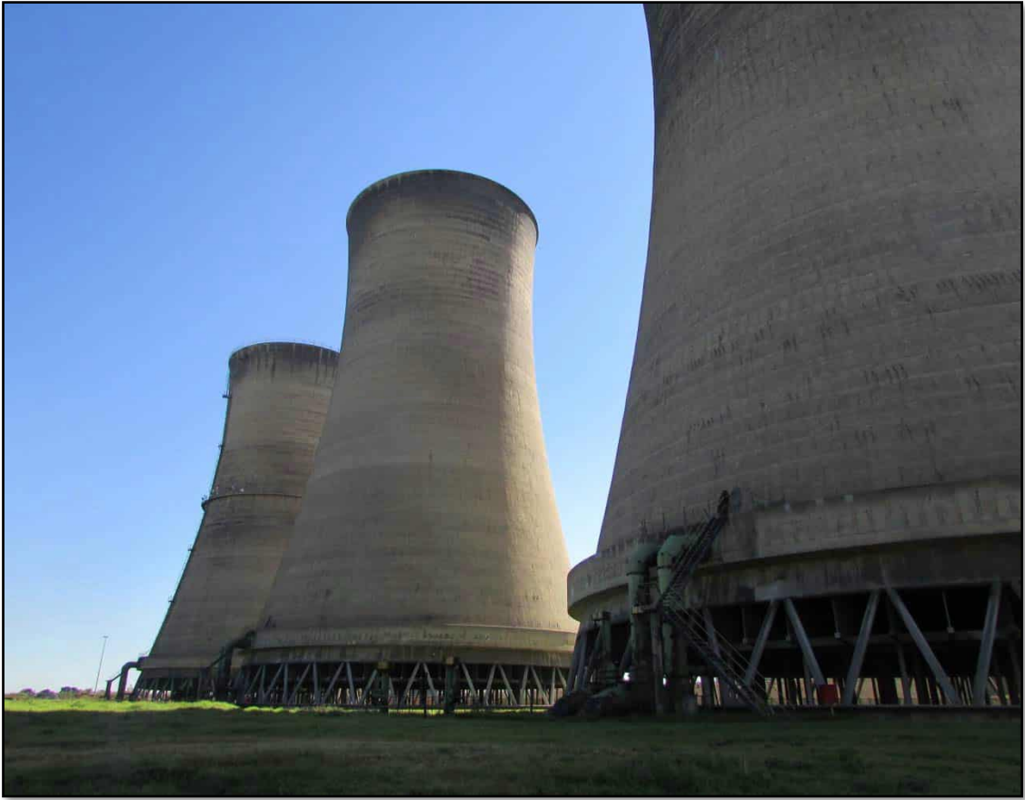
Figure 14: A view of A-Station's Cooling Towers.
