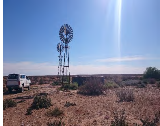
BH2 – wind pump
