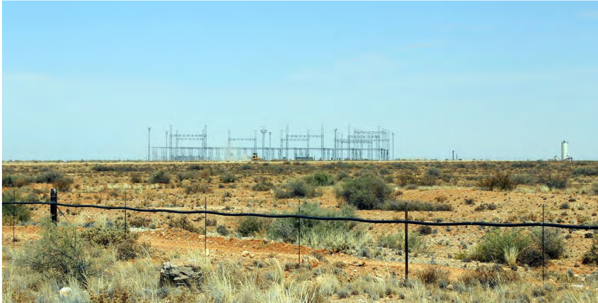
Figure 1-14 Eskom Nieuwehoop Substation currently under construction (Photo site SCA010)
