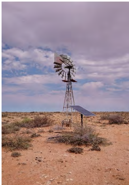
BH5 – wind pump
