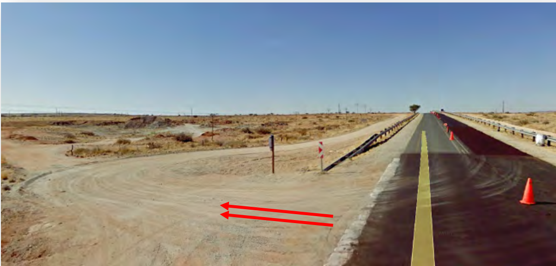
Photo 1: R27 towards the south (taken towards Kenhardt). The board shows “Loop 14”, located to the left, which is accessed via the Transnet Service Road. (Image source: Google, 2010)
