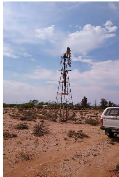
BH6 – wind pump
