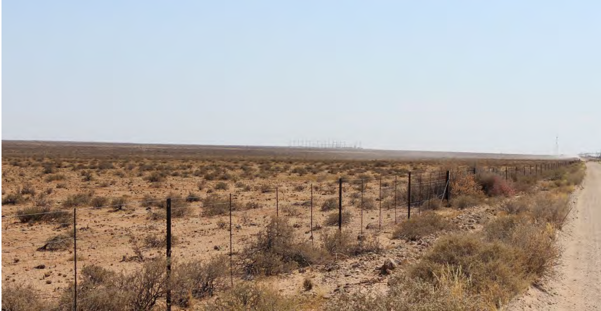
Figure 1-10 View north-west from viewpoint SCA04 along the proposed transmission line route. The new Eskom Nieuwehoop Substation is central in view and the tower at Rugseer Siding is to the right.
