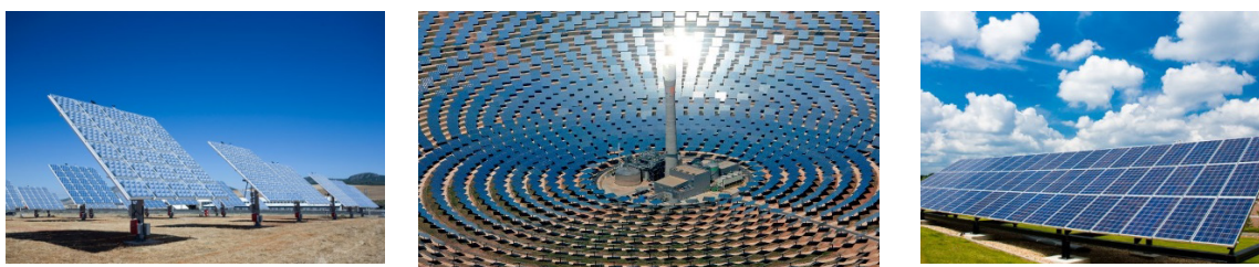
Figure 2.1: Solar panel technologies: CPV (left), CSP (middle) and conventional PV (right) 1
