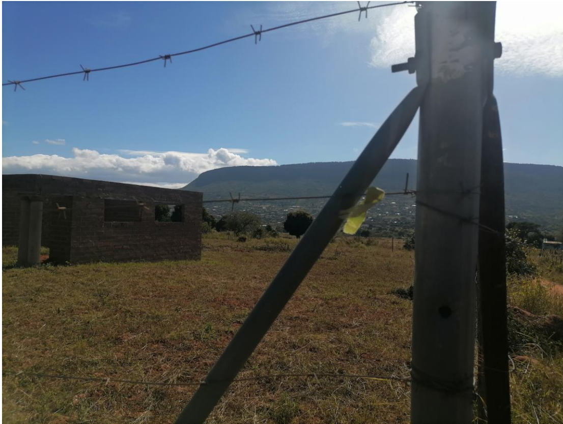
The peg on site
