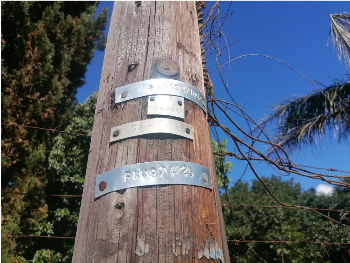
The existing pole number on site
