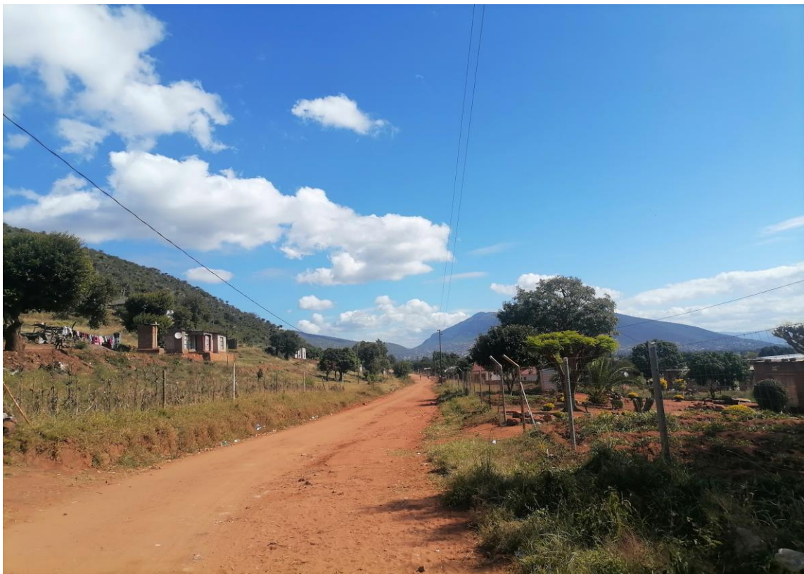
The existing powerlines and poles on site
