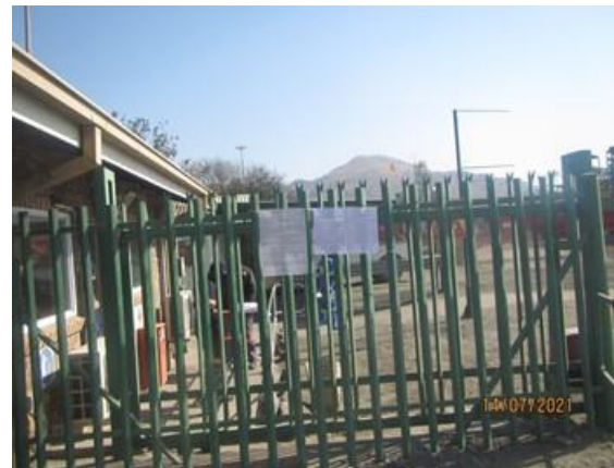
Plant Entrance (Project 4 and 5)
