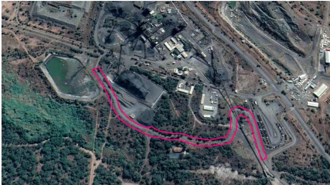
Figure 10: Widening of Access Road
