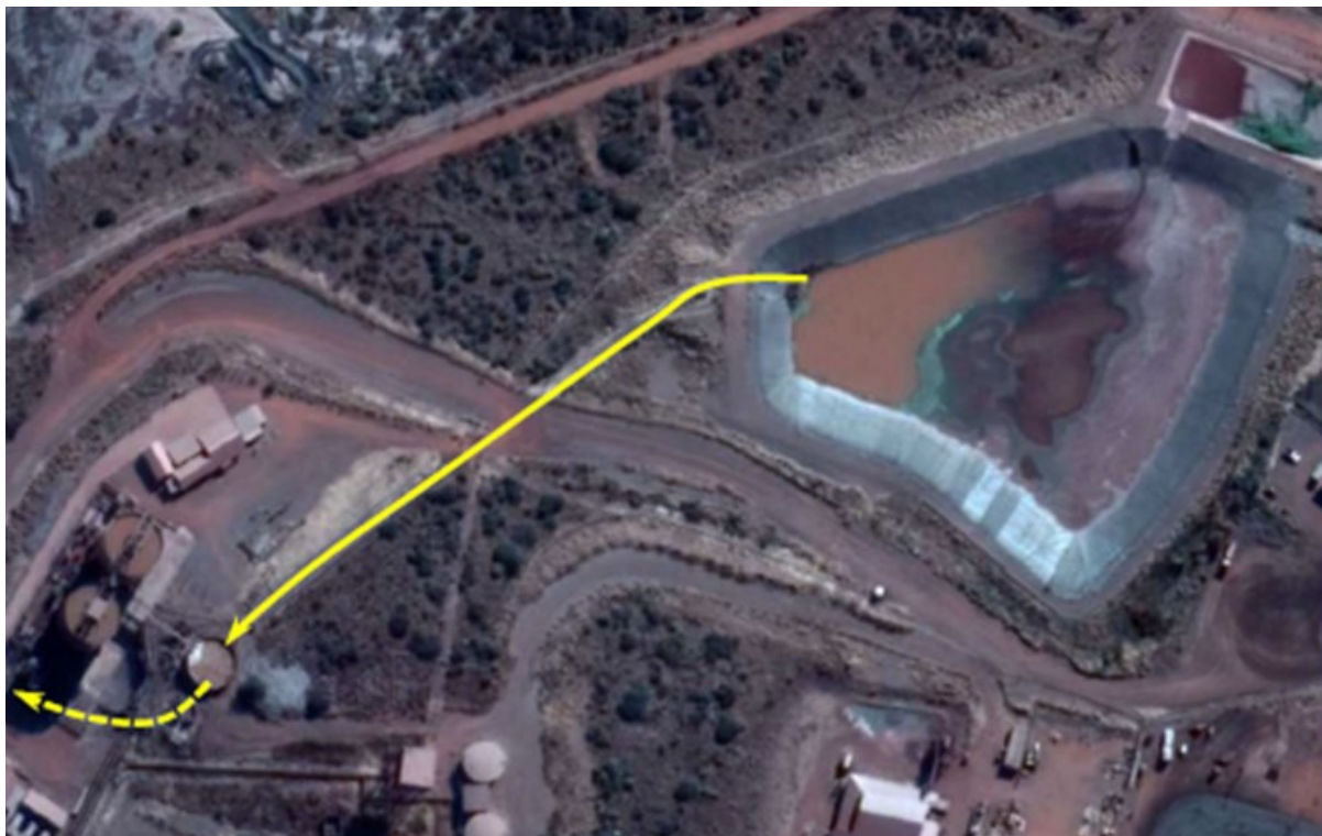
Figure 7: Location of the Thickener Tank and the Return Water Dam
