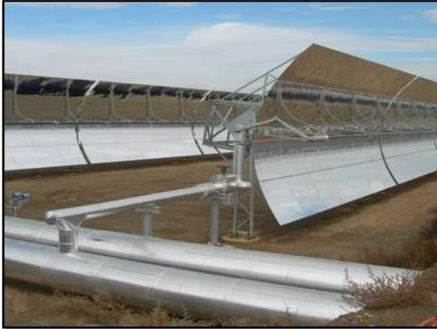
Figure 2: Parabolic trough solar collector assembly
