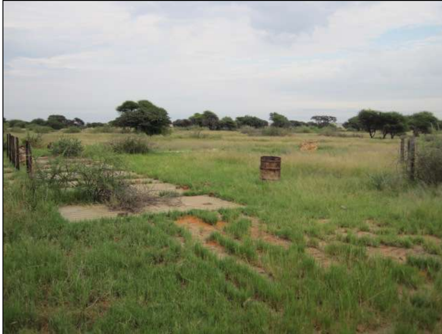
Figure 67: Site 4c cement foundations leading to the dip, Block 3.
