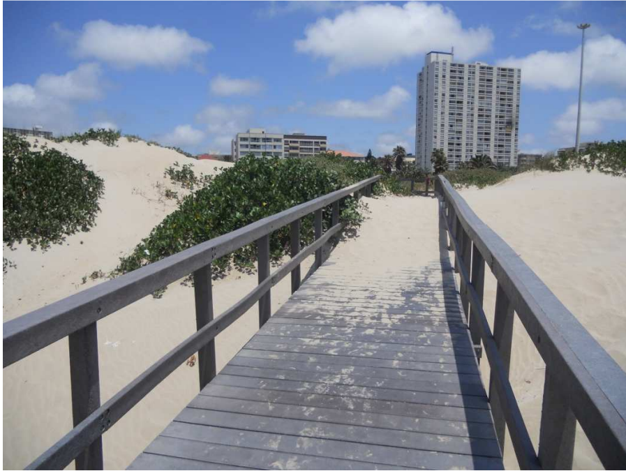
Figure 9: A view of an existing boardwalk in the area where Boardwalk 2 is proposed.
