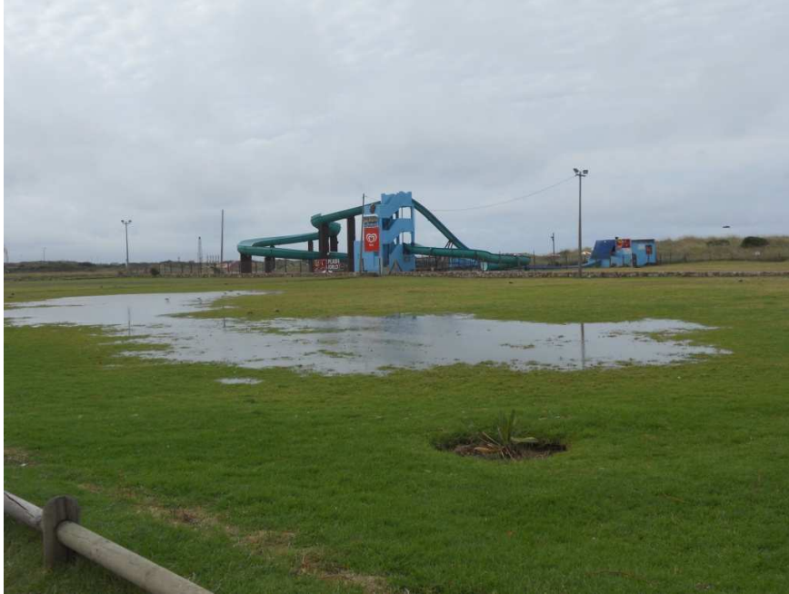
Figure 1: A view of the area in front of the Supertubes after heavy rainfall.
