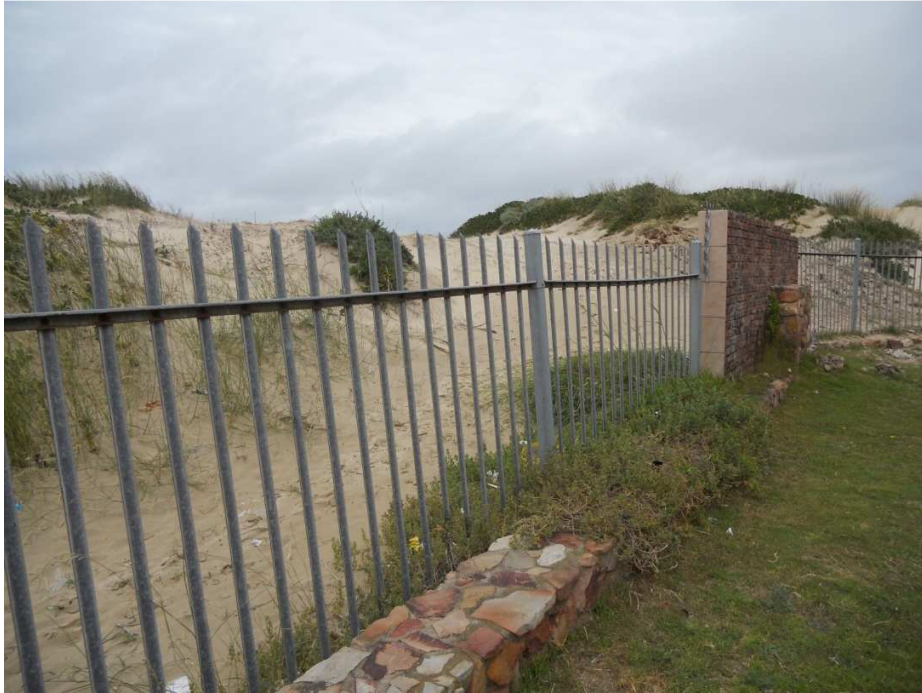
Figure 5: The area directly adjacent to the fence on the beach side was a constructed paved path 6 months prior to this photo.
