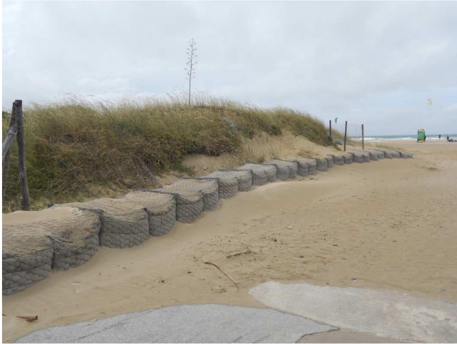
Figure 3: A view of the access to the beach on the seaward side. Note attempts that have been made to prevent erosion and stabilize dunes using sandbags.
