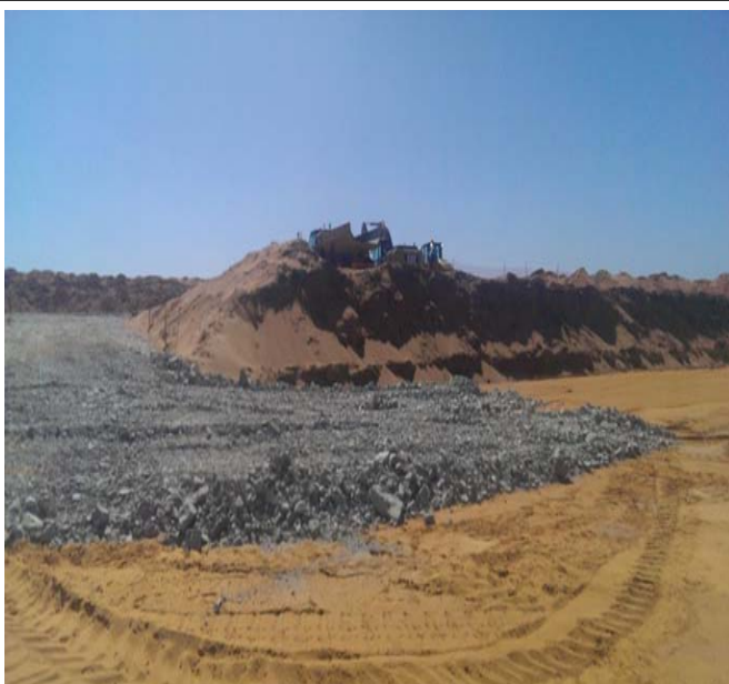
Photograph 7.3: Construction of terrace and foundations for substation (Sere Wind Facility)
