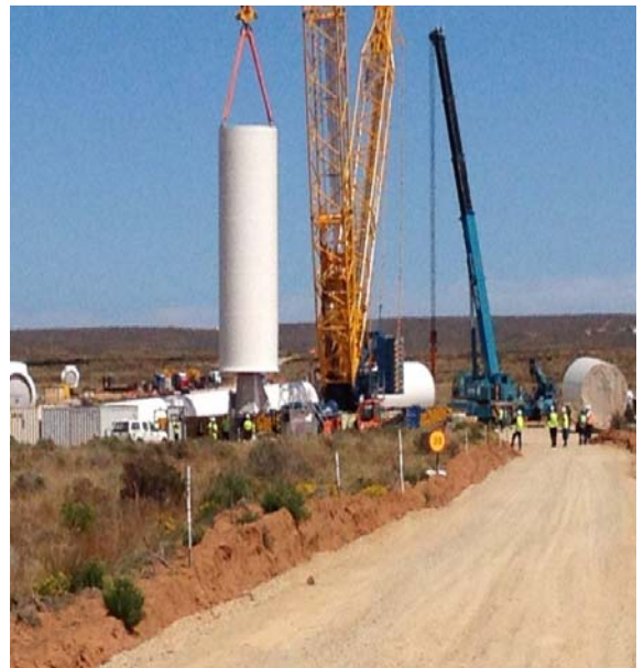
Photograph 7.2: Tower sections being lifted (Sere Wind Facility)
