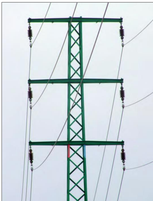
conductors slung below the support arms
