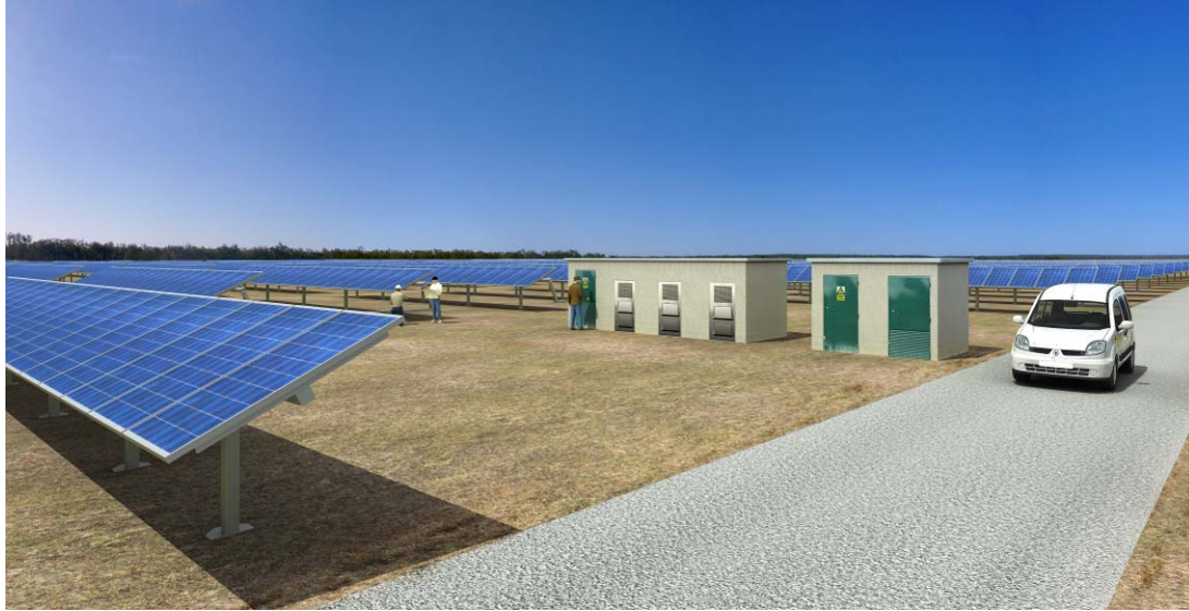
Figure 2.4: Conceptual drawing showing an inverter cabins (Courtesy of Acciona)
