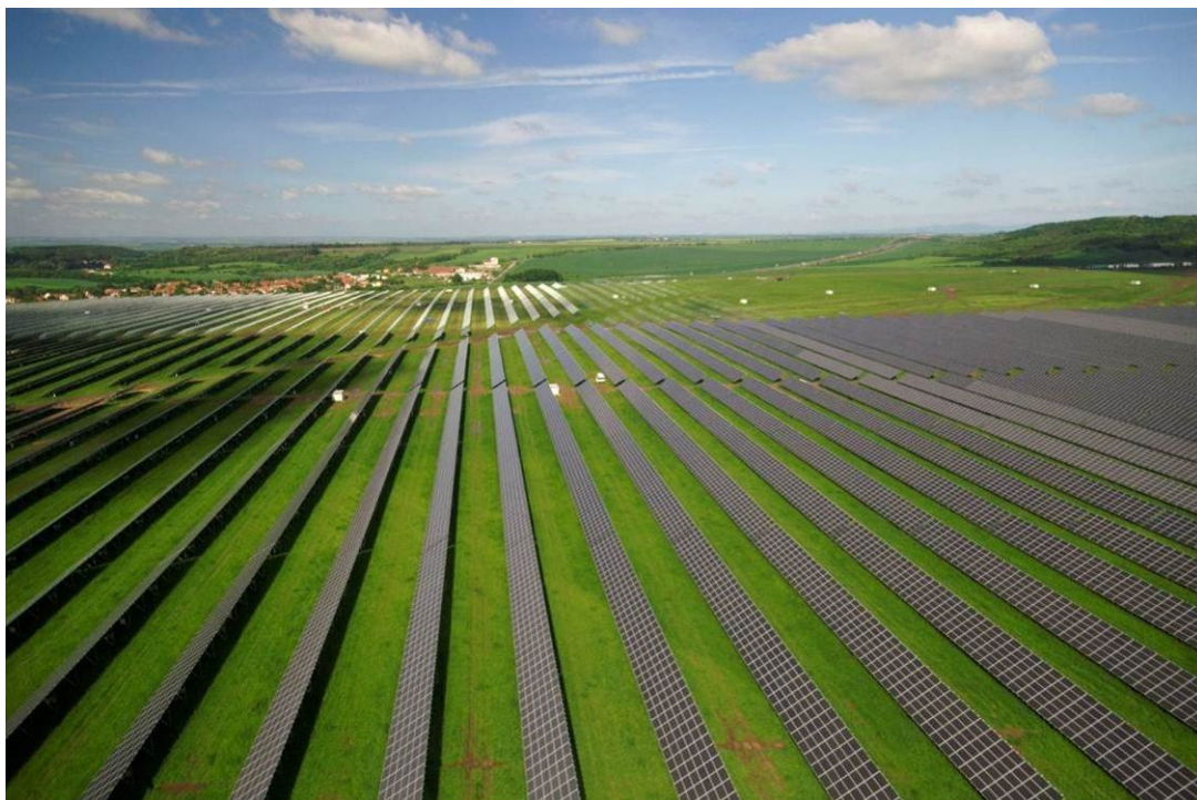
Figure 2.5: Illustration of a photovoltaic solar facility (Courtesy of Decchi)
