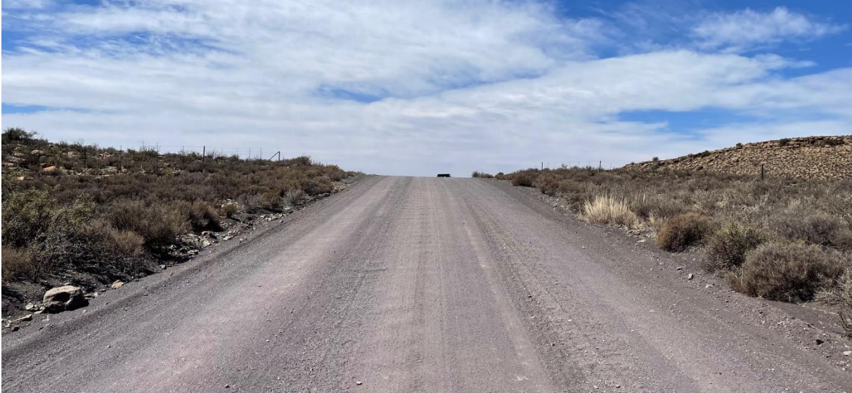
Figure 7-10 Vertical Curve at Km 89.55 on Road DR2312 with a vehicle in the background
