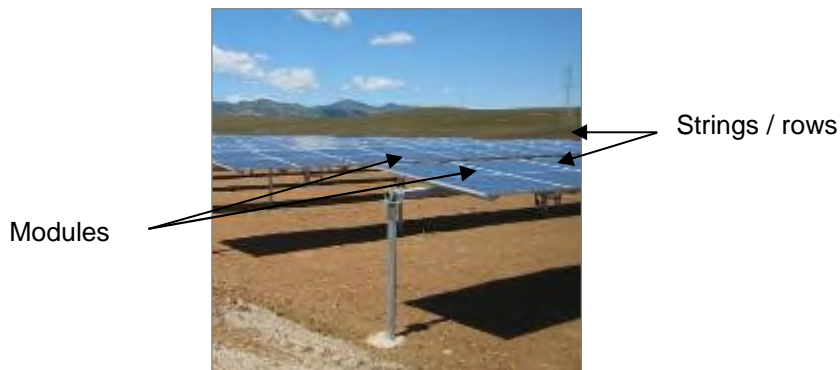
Figure 2.2: Typical layout of panel structures
