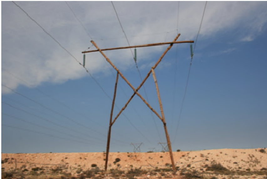
Figure 2.1: Example of an existing 132 kV transmission line onsite (taken 29/09/2011)
