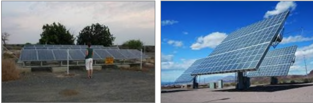
Figure 2.8: Photovoltaic solar cells (left) 23 and a CPV system (right) 24 were considered for the proposed PV plant
