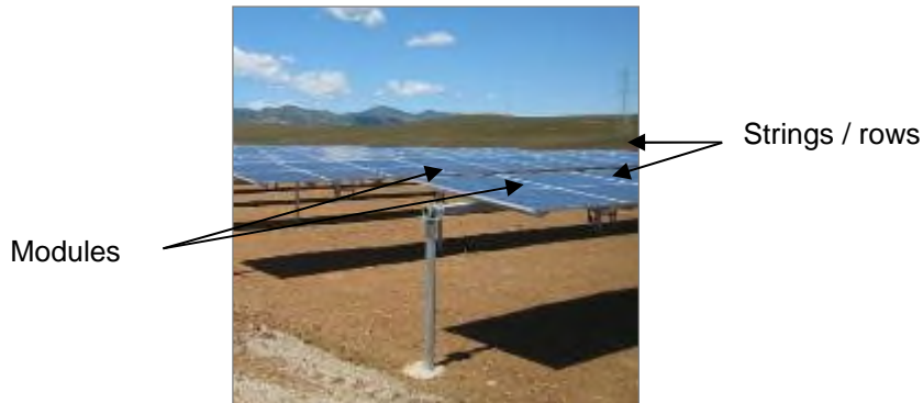
Figure 2.3: Typical layout of panel structures
