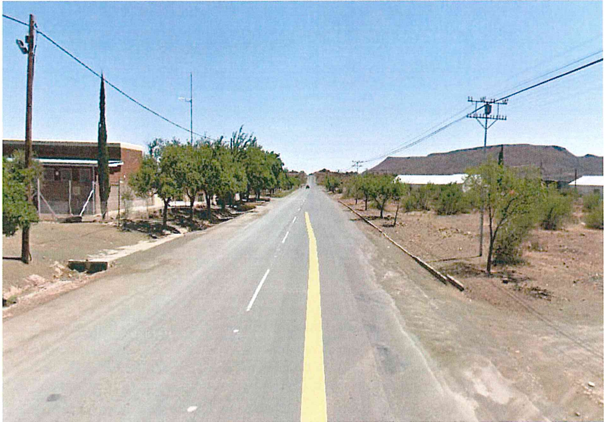
Photo 9: Northern view of Provincial Main Road (R48) through northern residential areas of Petrusville. Note the sedimentation on the road surface due to overland storm water run-off.
