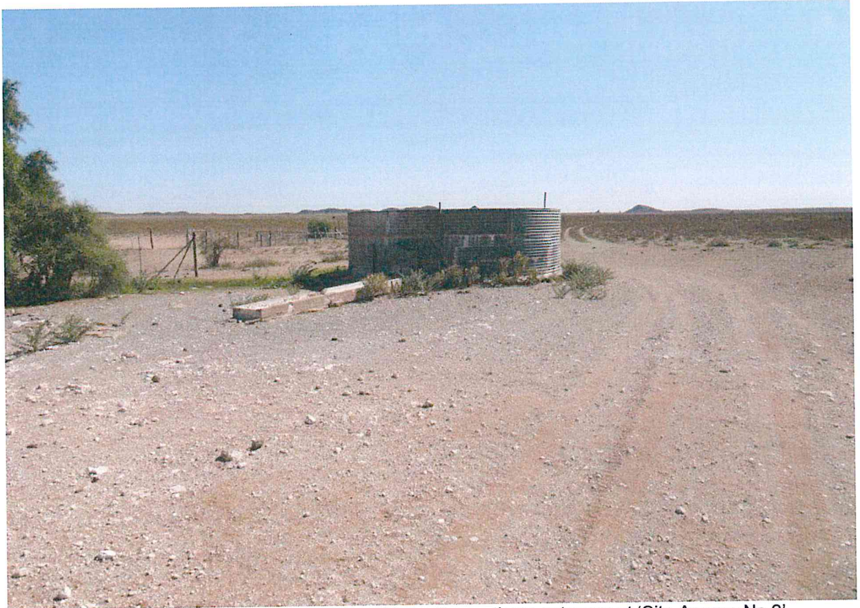
Photo 18: View of the Kalkpoort Road from the northern entrance at 'Site Access No.2'. Note the narrow two-track path and open flat topography available to upgrade the existing road
