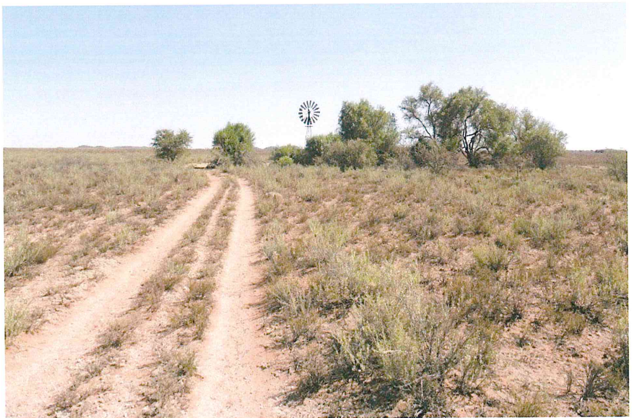
Photo 17: View of the Kalkpoort Road from the northern entrance at 'Site Access No.2'. Note the narrow two-track path and open flat topography available to upgrade the existing road.
