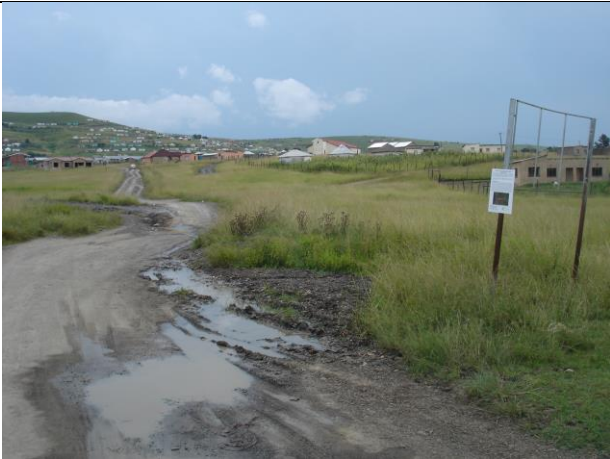
Figure 1. Image showing existing cemetery site access road adjoining the R56 road.
