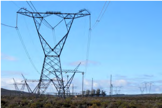
Existing powerlines and substation to the south of the site
