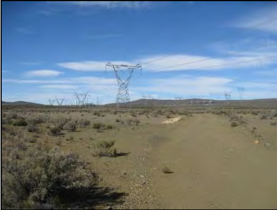
Photograph 1.4: Eskom Komsberg substation located adjacent to Saaiplaas farm
