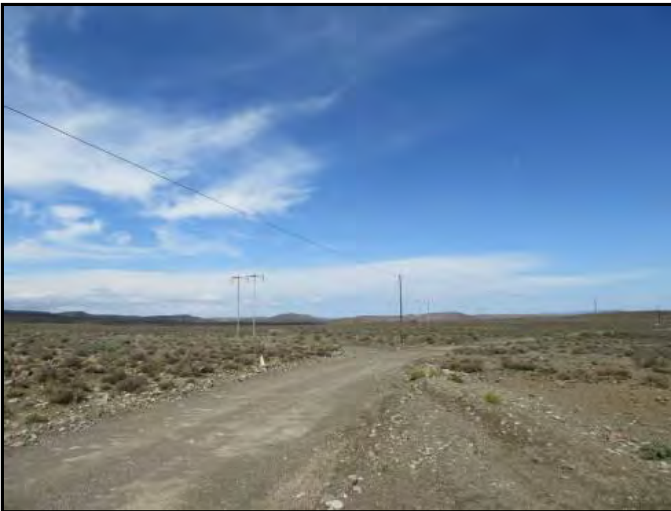
Photograph 1.17: Approximate location of proposed Tx line crossing of the Koornplaats-Komsberg gravel road south of Wilgerboom farmstead
