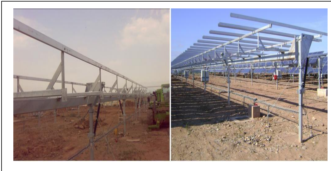
Figure 3.4: Frame, structural details (Courtesy of Igeam, 2011)
