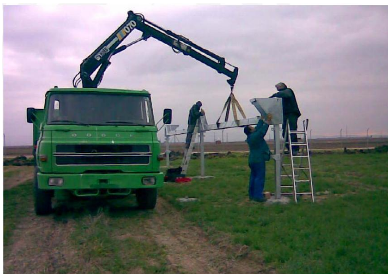
Figure 3.5 Mounting of the frame for the PV panels (Courtesy of Igeam, 2011)
