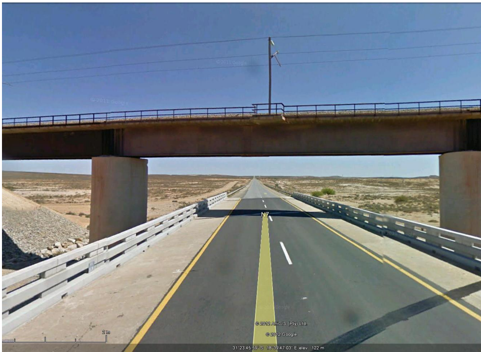
Overhead Railway Bridge on N7, Vanrhynsdorp
