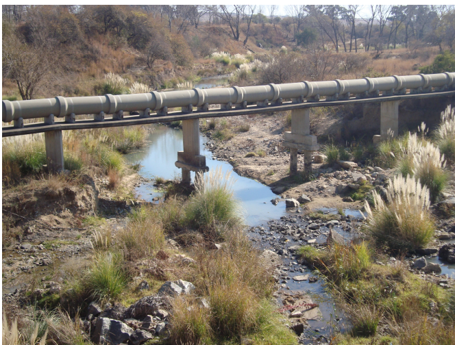
Figure 1: Pipe bridge supporting the sewage pipeline to Sunderland Ridge
