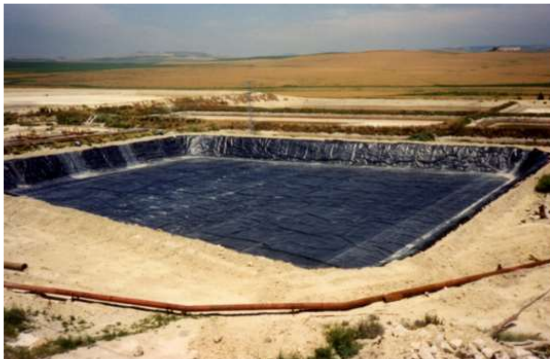
Figure 3.6: Photograph of a typical lined evaporation pond utilised for a CSP Project
