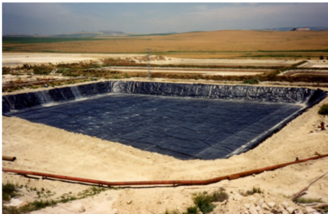
Figure 4.7: Photograph of a typical lined evaporation pond utilised for a CSP Project
