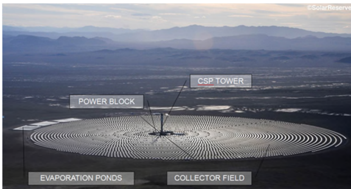
Figure 4.4: Photograph illustrating a constructed SolarReserve South Africa CSP Facility, Crescent Dunes, located in Tonopah, Nevada (courtesy of SolarReserve South Africa)
