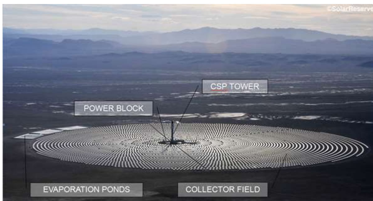
Figure 4.4: Photograph illustrating a constructed SolarReserve South Africa CSP Plant, Crescent Dunes, located in Tonopah, Nevada (courtesy of SolarReserve South Africa)
