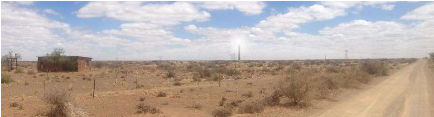
Figure 8.7: Post construction panoramic view from a ~5km distance from the tower
