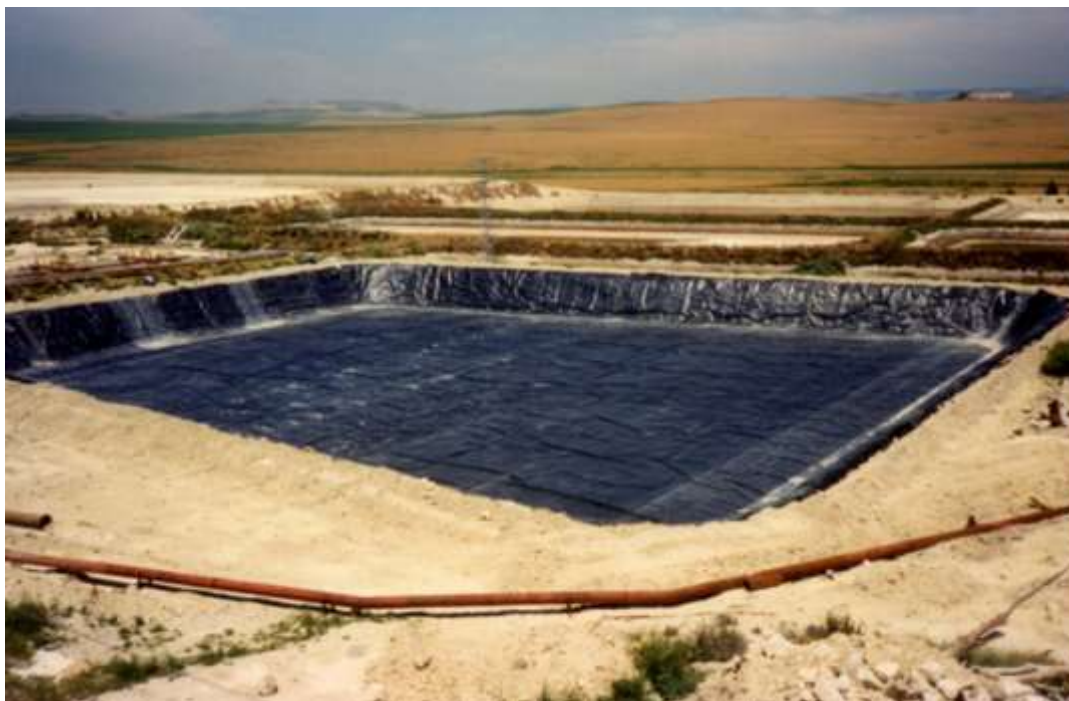
Figure 4.7: Photograph of a typical lined evaporation pond utilised for a CSP Project
