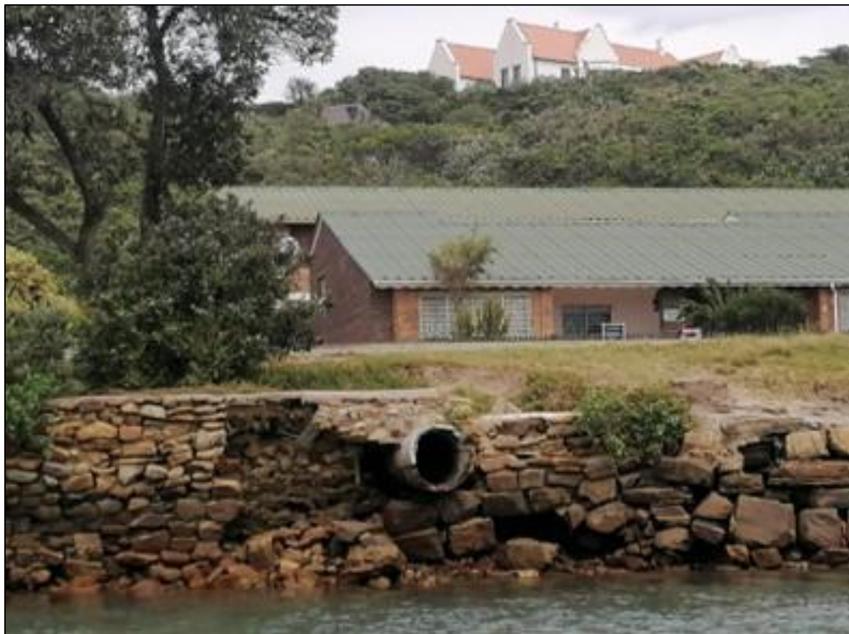
Figure 3.4: Stormwater pipeline outlet located near the mouth of the Kowie Estuary.
