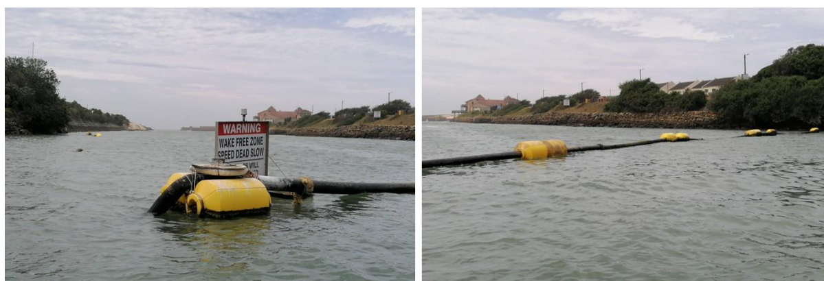
Figure 3.16: Dredge pipeline observed within the Kowie Estuary mouth.
